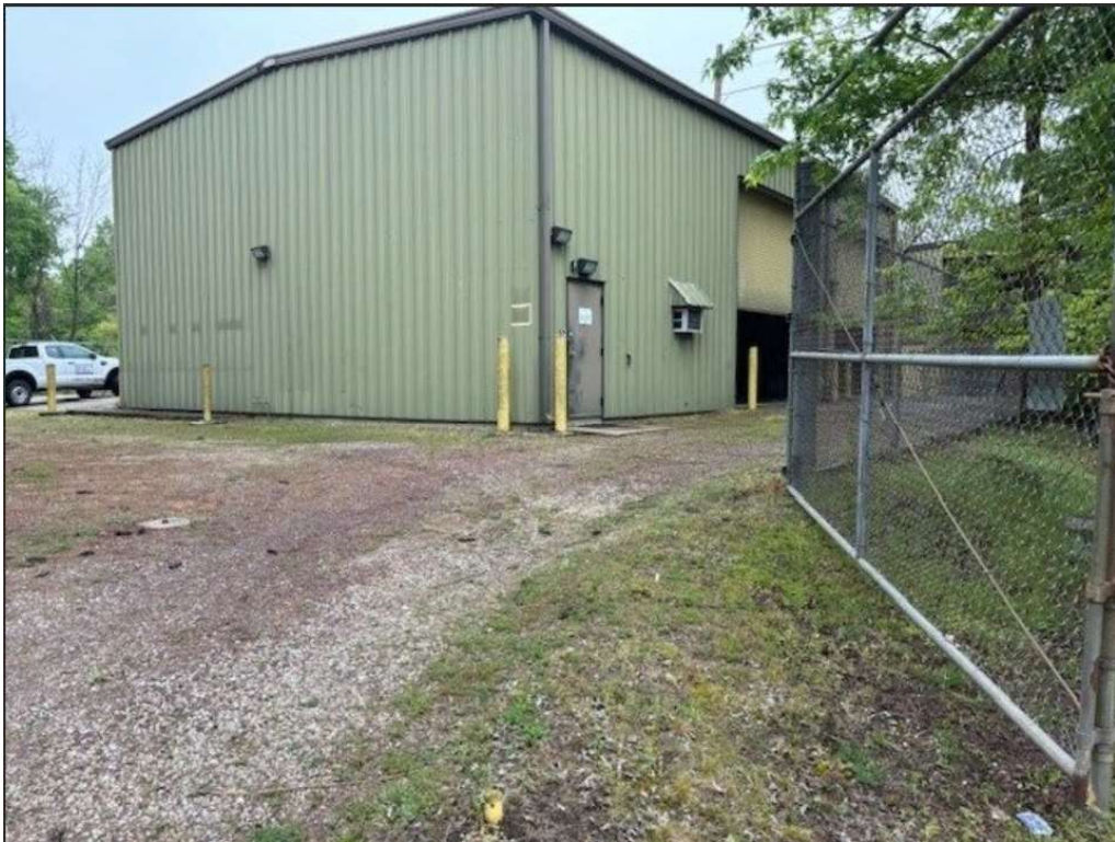
Ground water treatment plant
