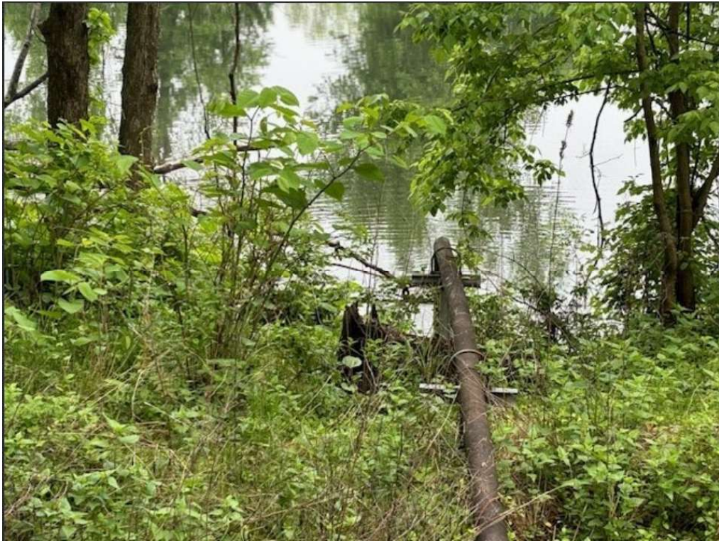
Effluent discharge to the Schuylkill River
