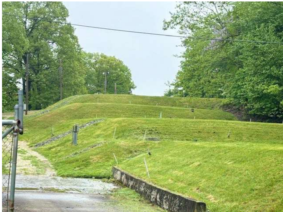
Terraced wet cap over lagoon area
