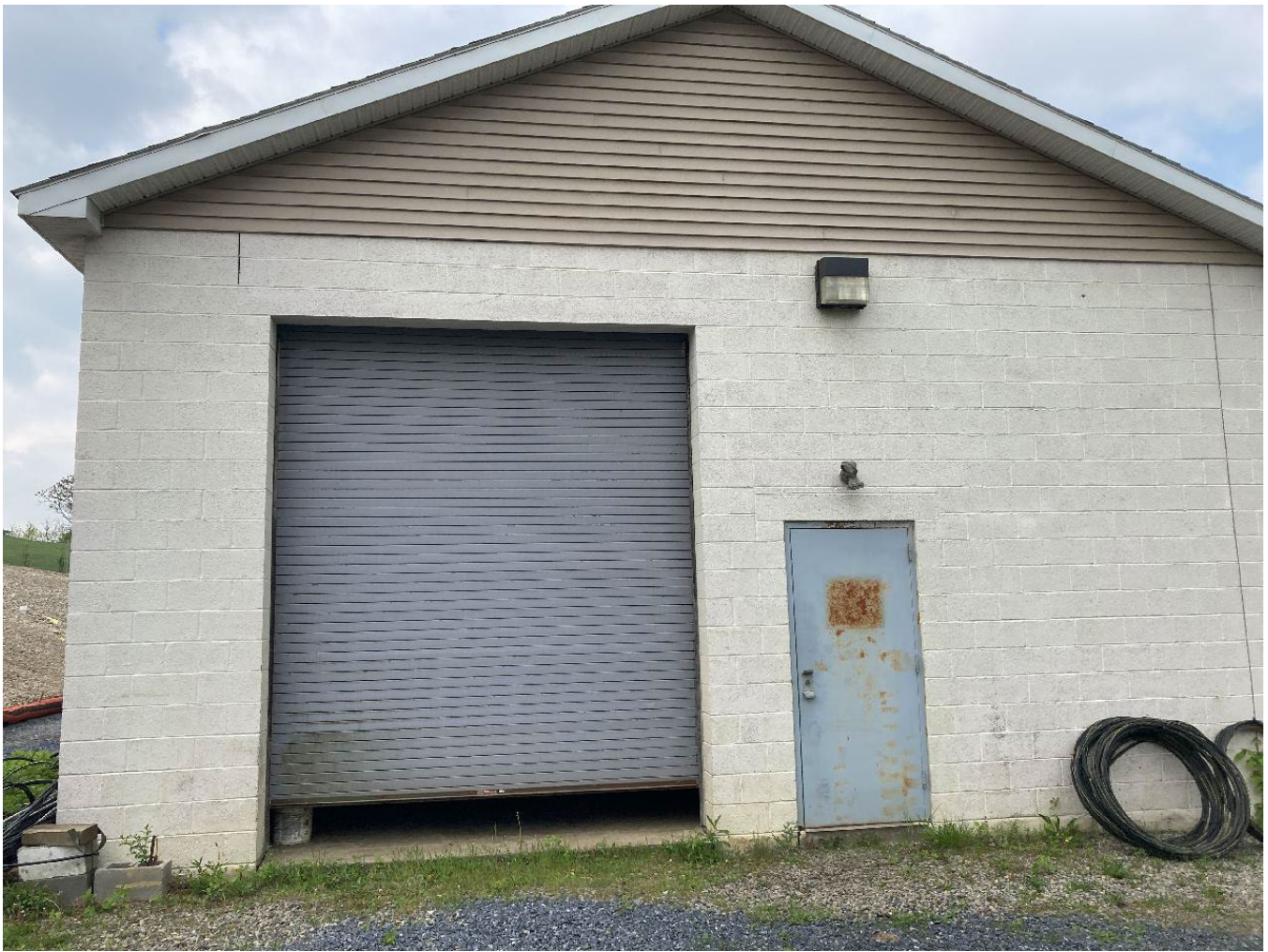
Water treatment building
