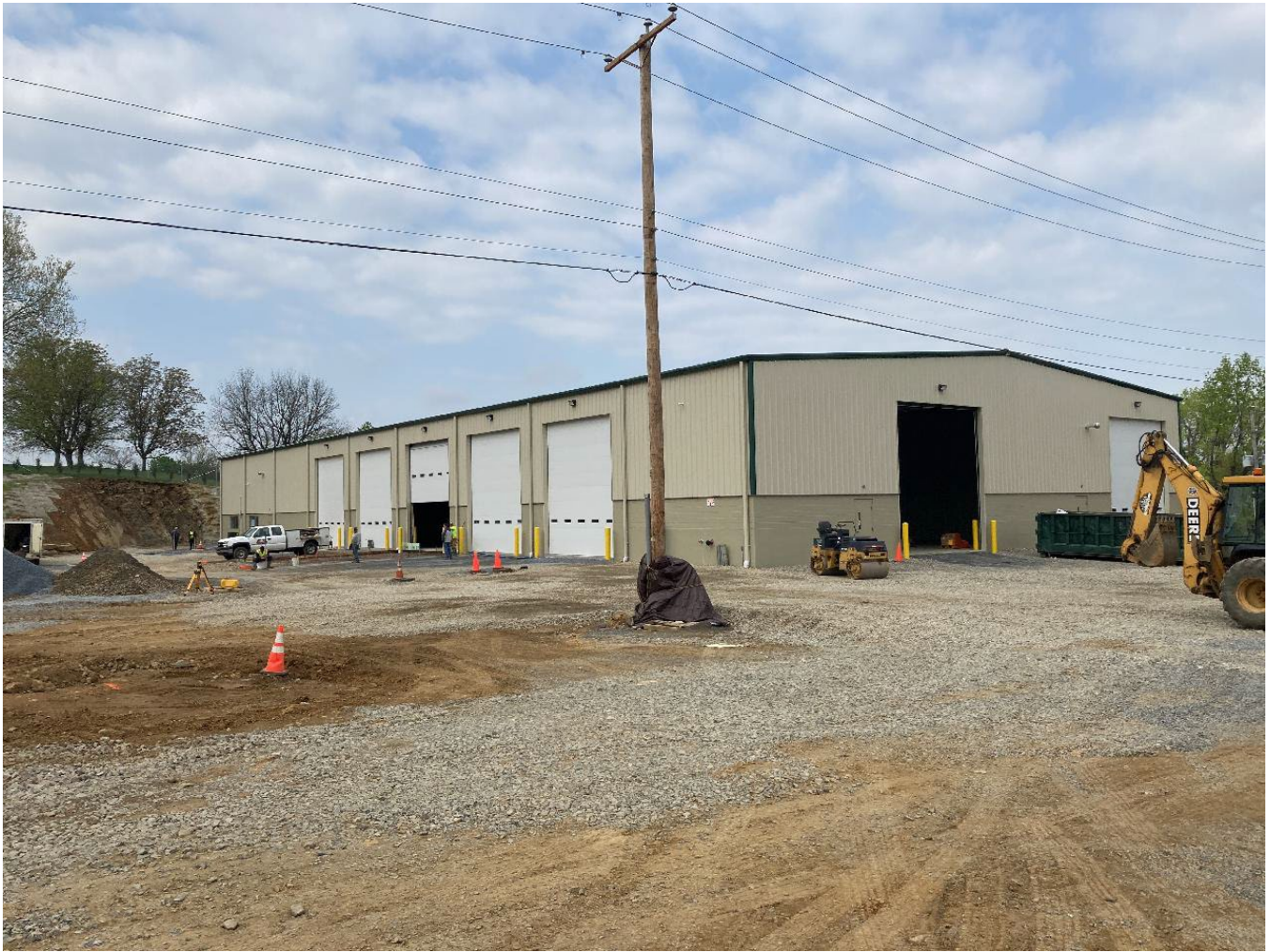
New Chrin warehouses near water treatment plant
