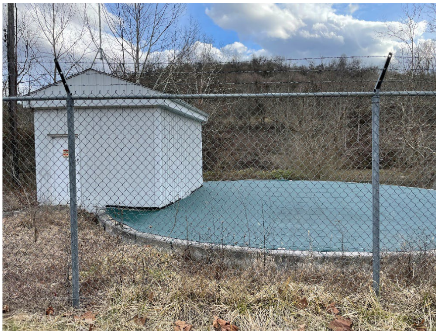
Pond 6 pumping station
