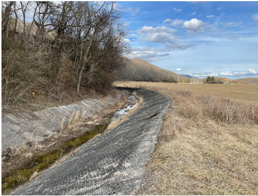
Western diversion ditch (facing northeast)
