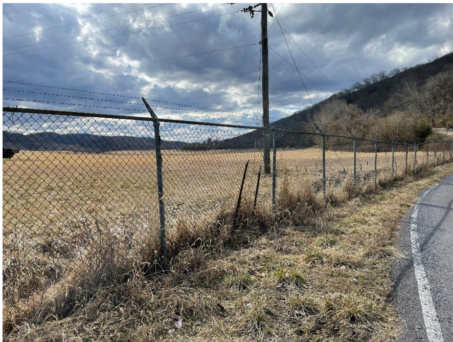
Fence along Route 611
