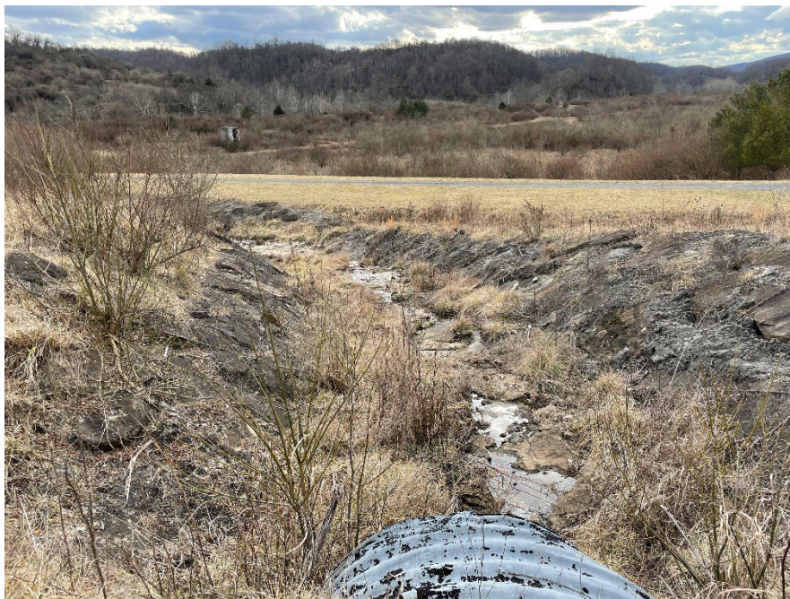
Western diversion ditch (facing southwest)
