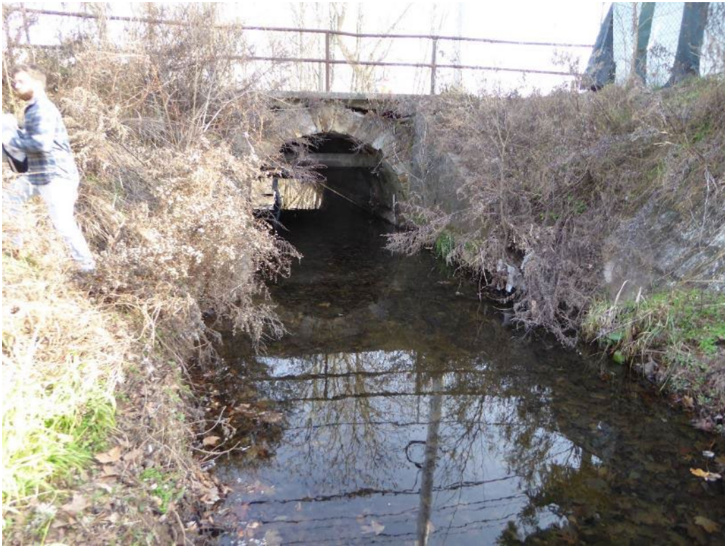
Tannery Run and Maple Street bridge
