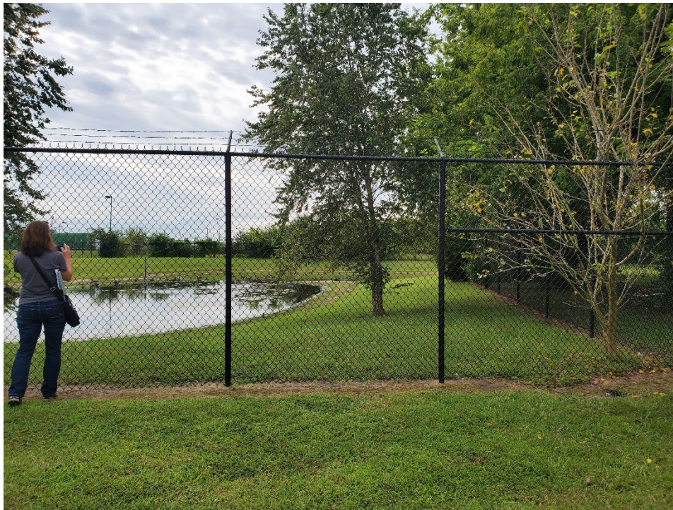
Stormwater Detention Basin on Race St.
