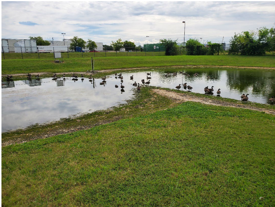
Stormwater Detention Basin on Race St.
