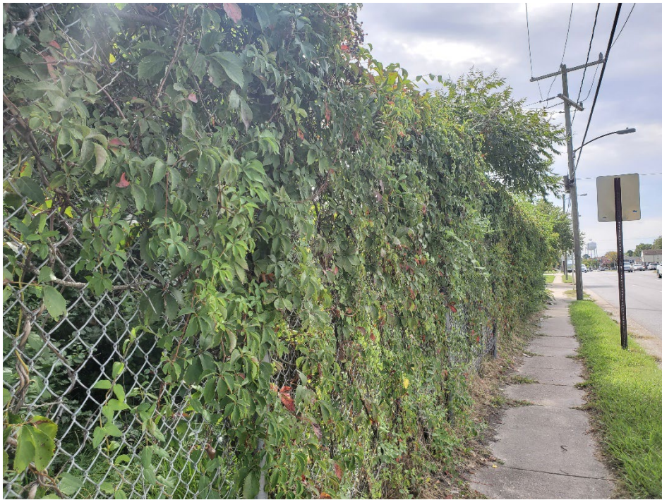
Fence along Effingham Street looking south
