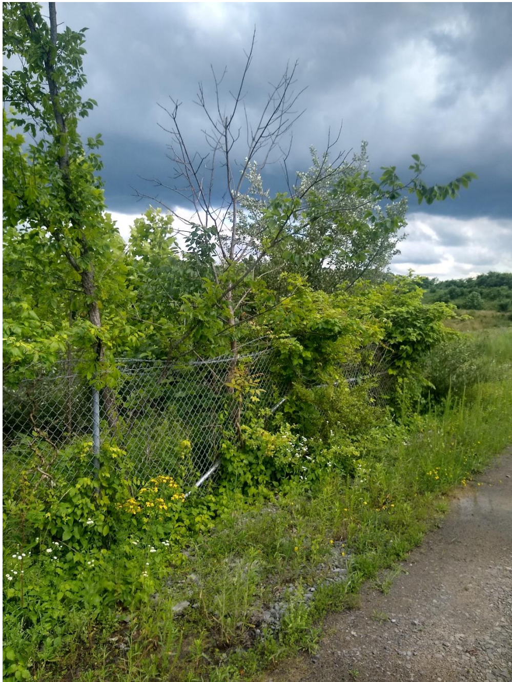
Damage to perimeter fence from fallen woody vegetation
