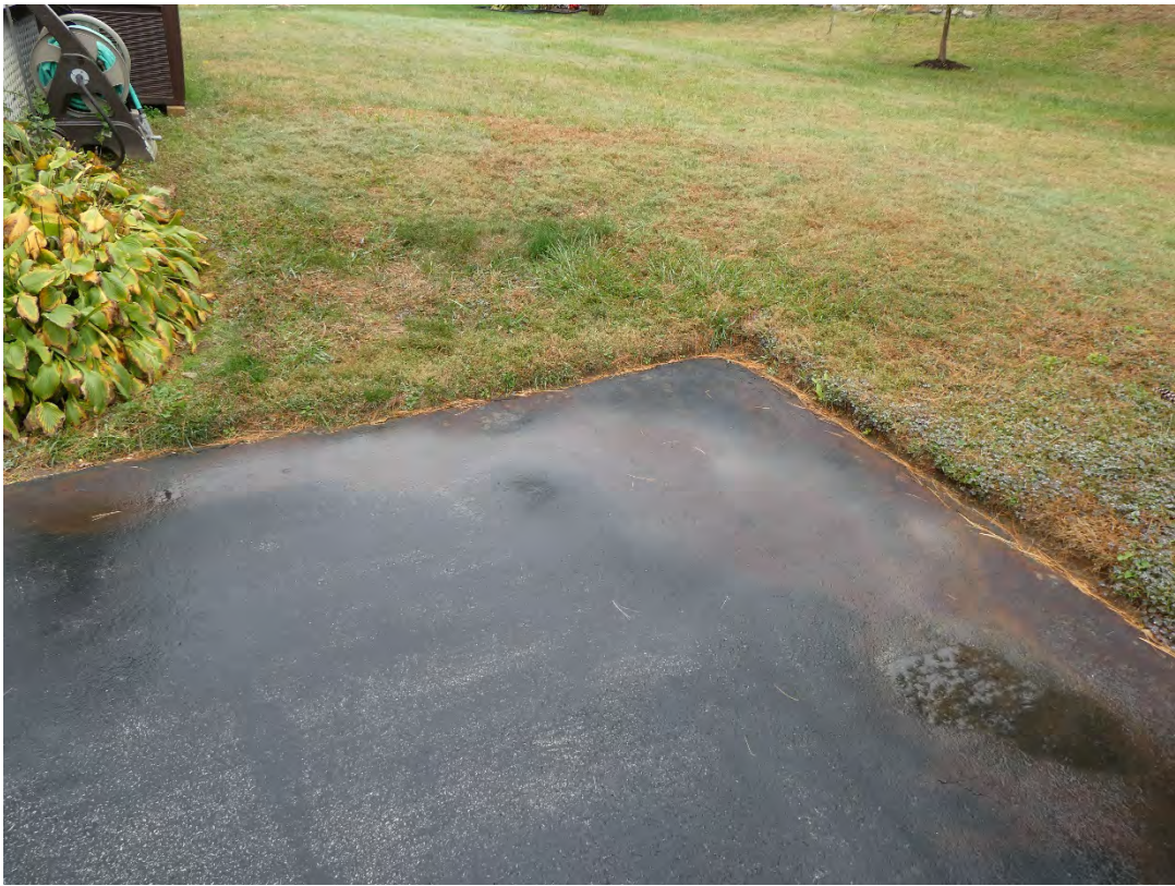
Staining in driveway from seep behind house on Rittenhouse Circle
