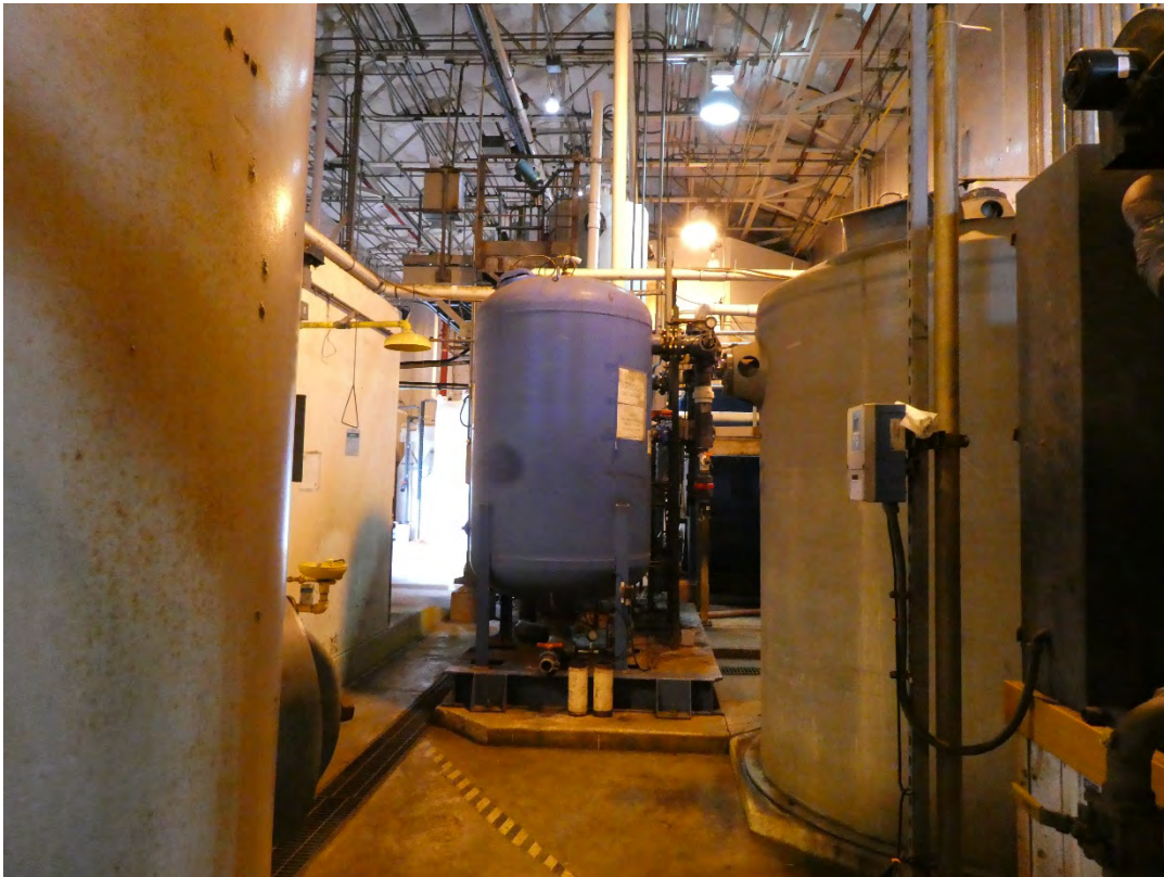
Inside treatment plant
