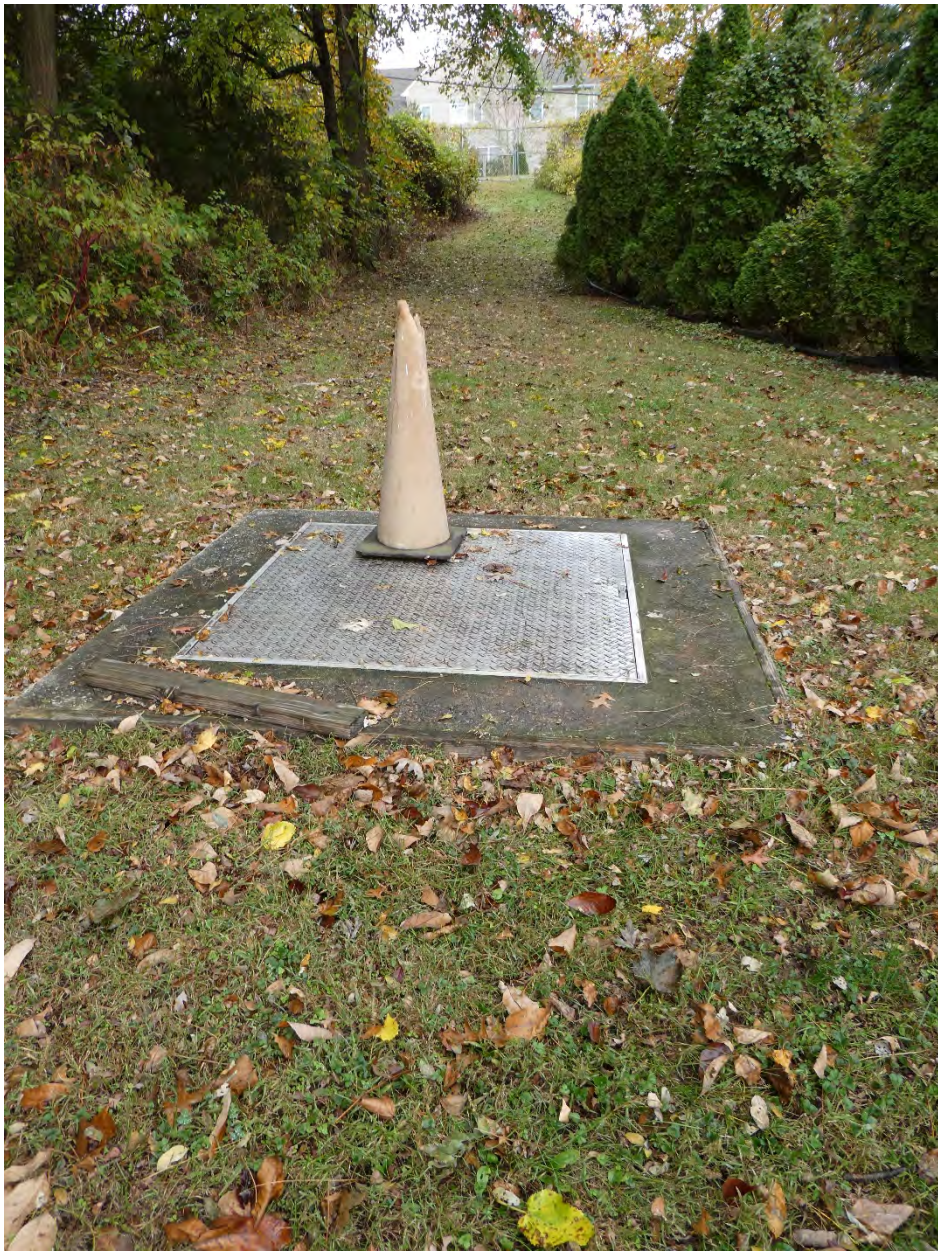
CTR sump in CTR area
