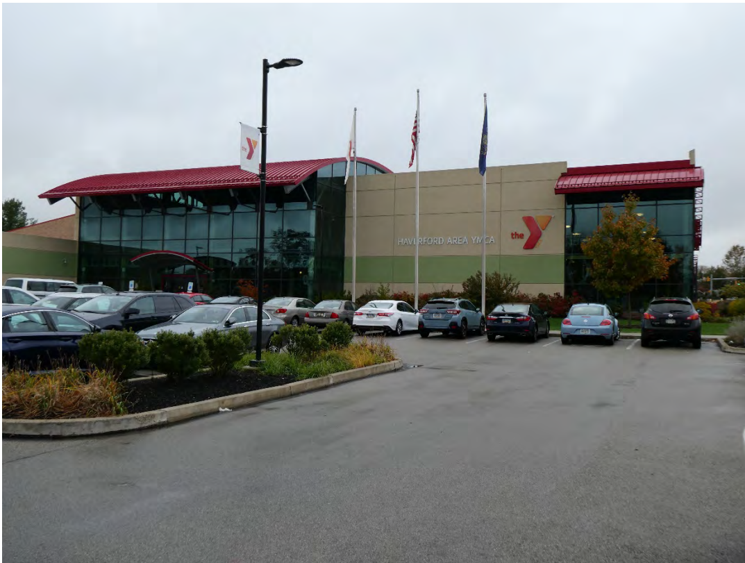
Haverford Area YMCA where PCG factory used to be
