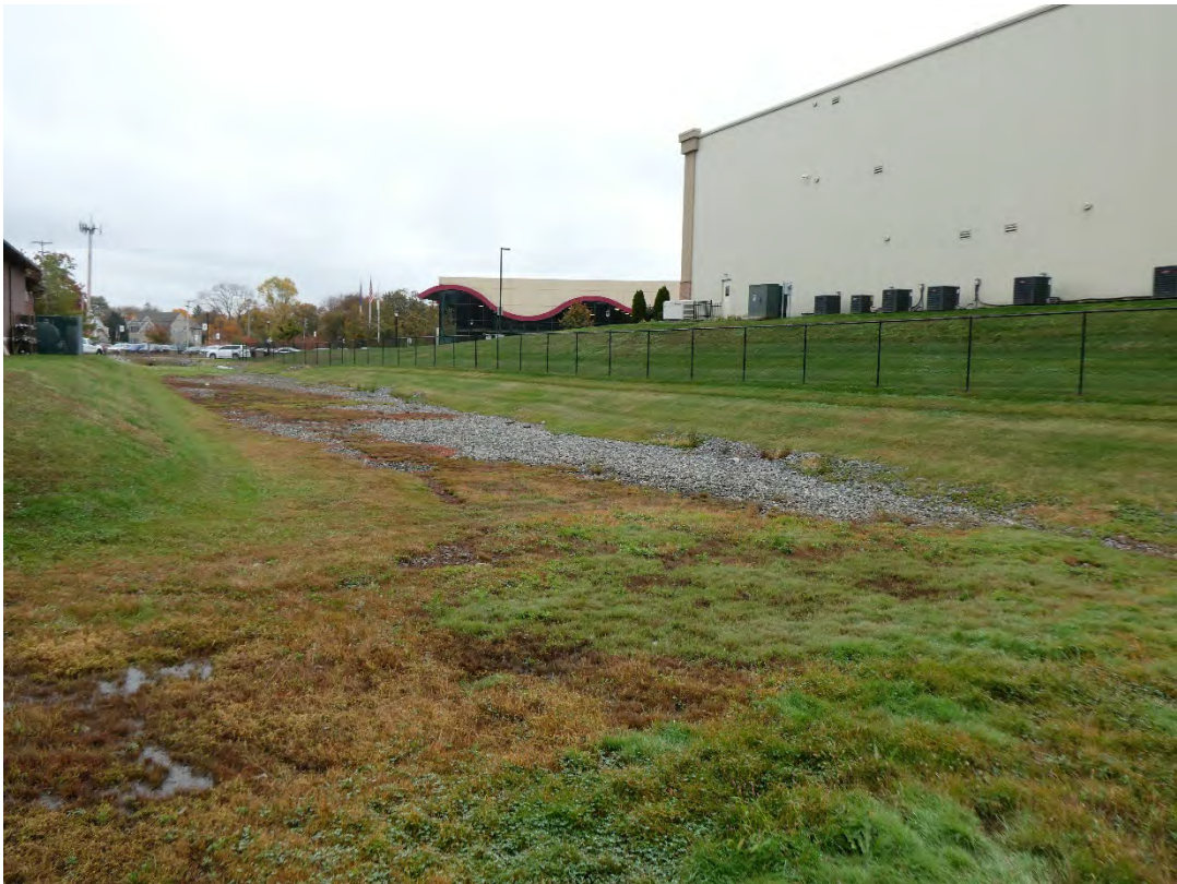
Catch basin between treatment plant and Mr. Storage facility with YMCA in background
