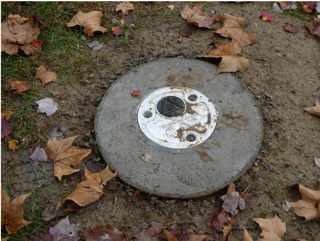
New well CW-35S behind house on Rittenhouse Circle
