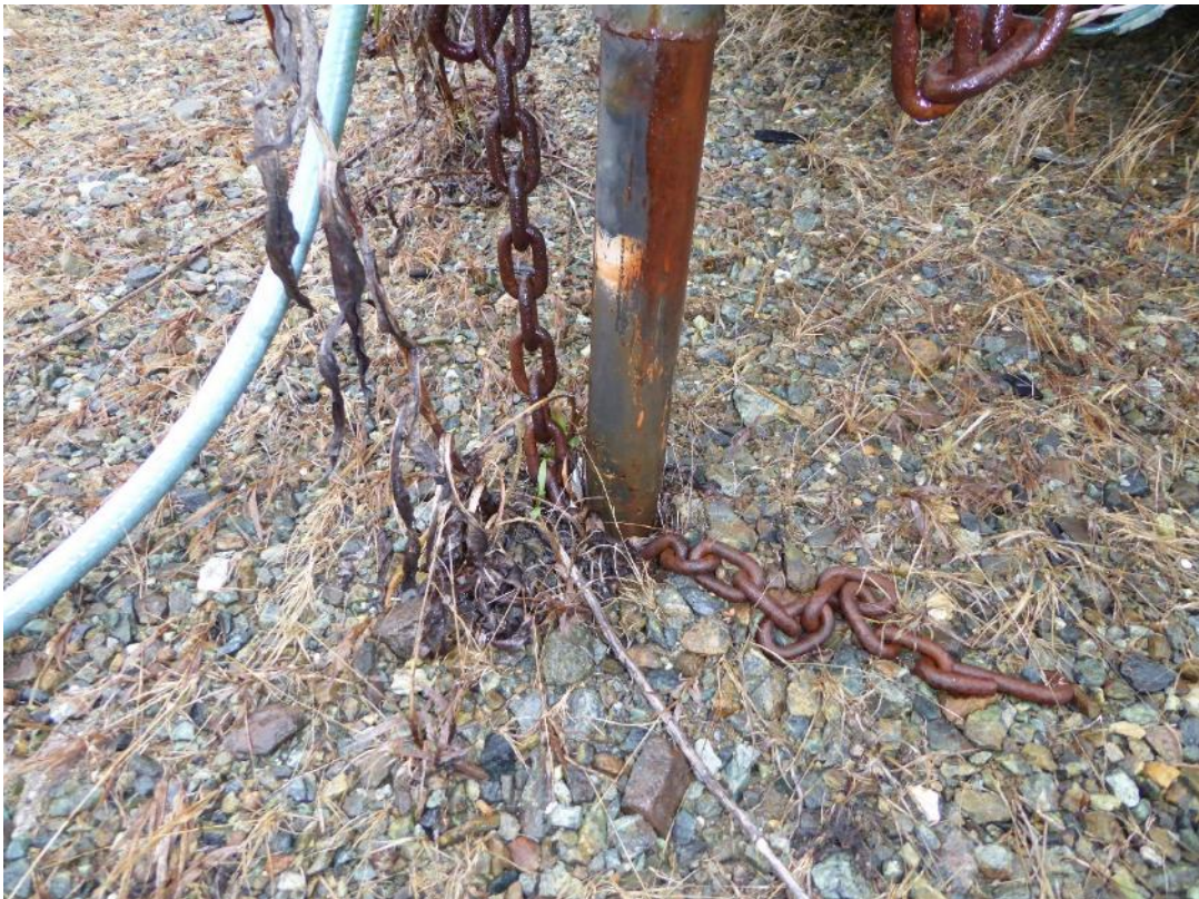
Trailer post sinking into cap at SBA
