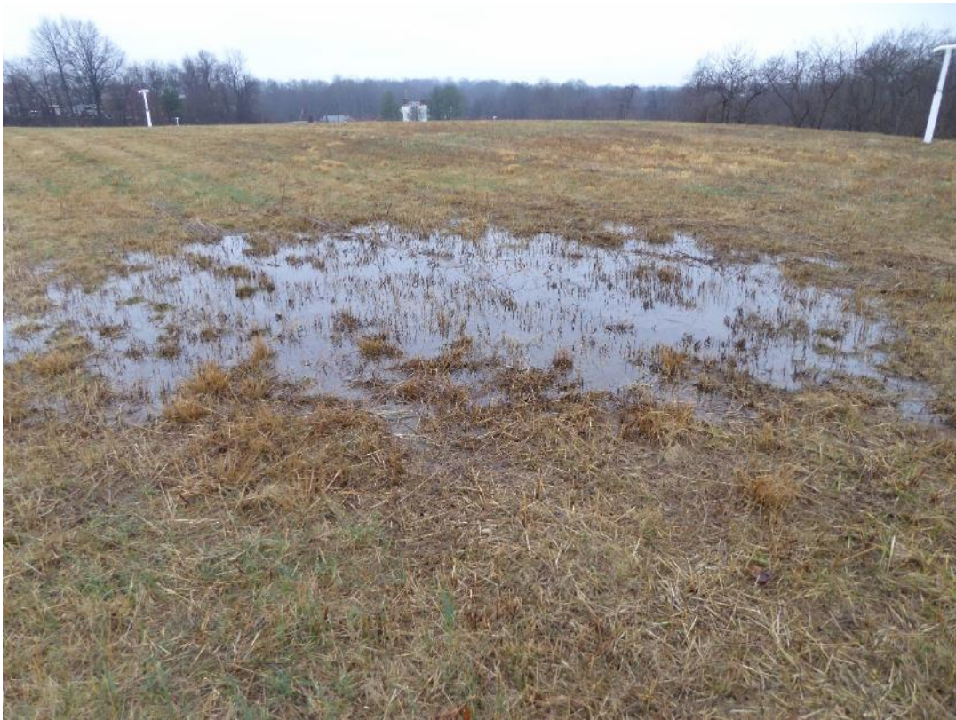
Ponding on Inert Area vegetated cap
