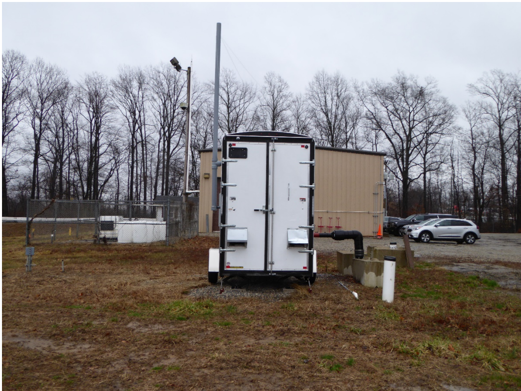
Trailer housing landfill gas extraction system blower and direct venting stack
