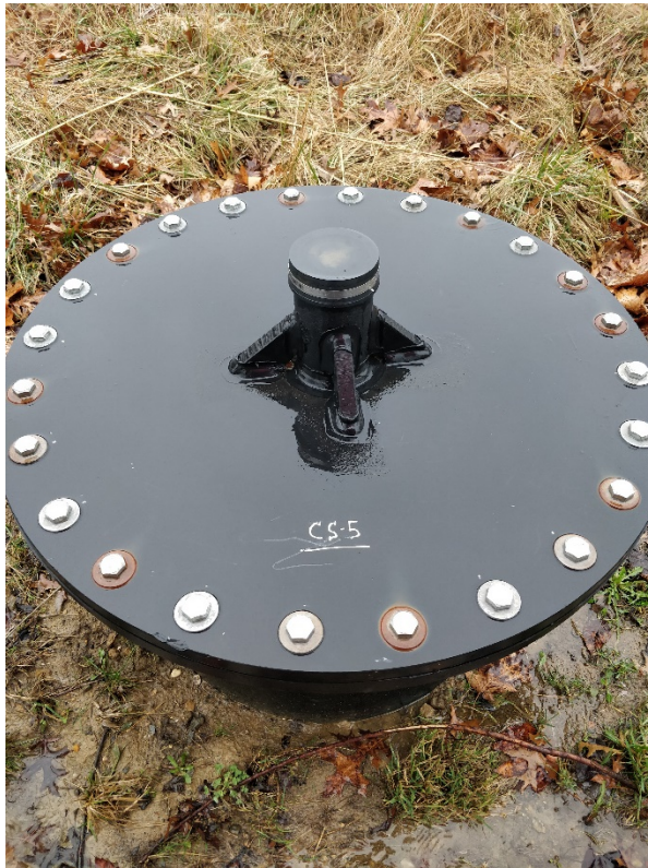
Landfill gas extraction system condensate sump
