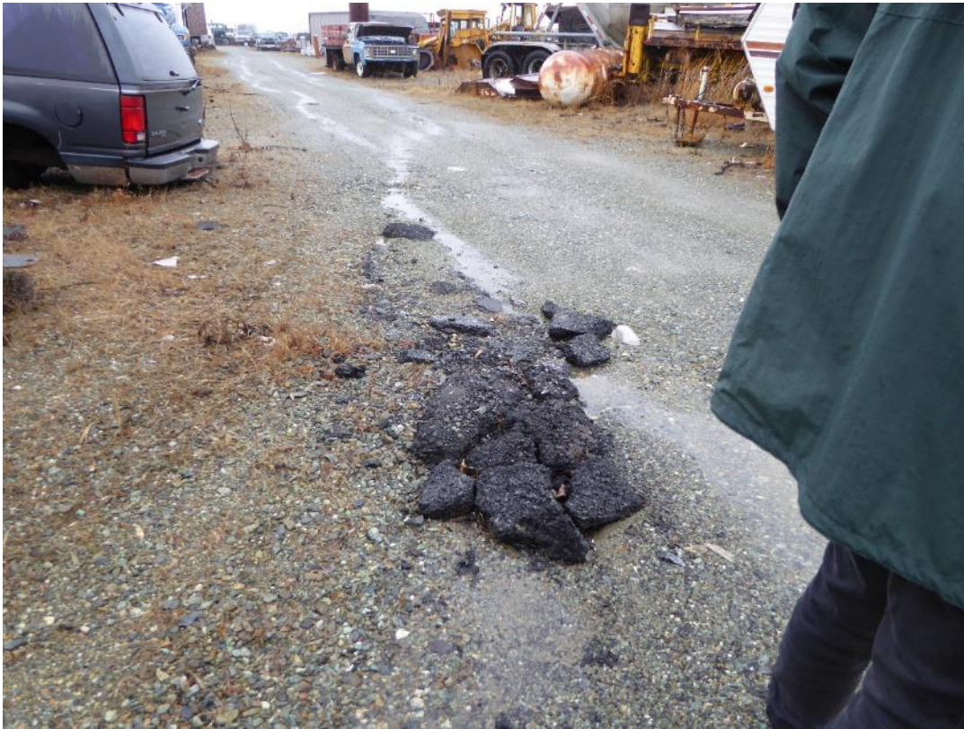
Asphalt chunks placed in rivulet on SBA to mitigate erosion
