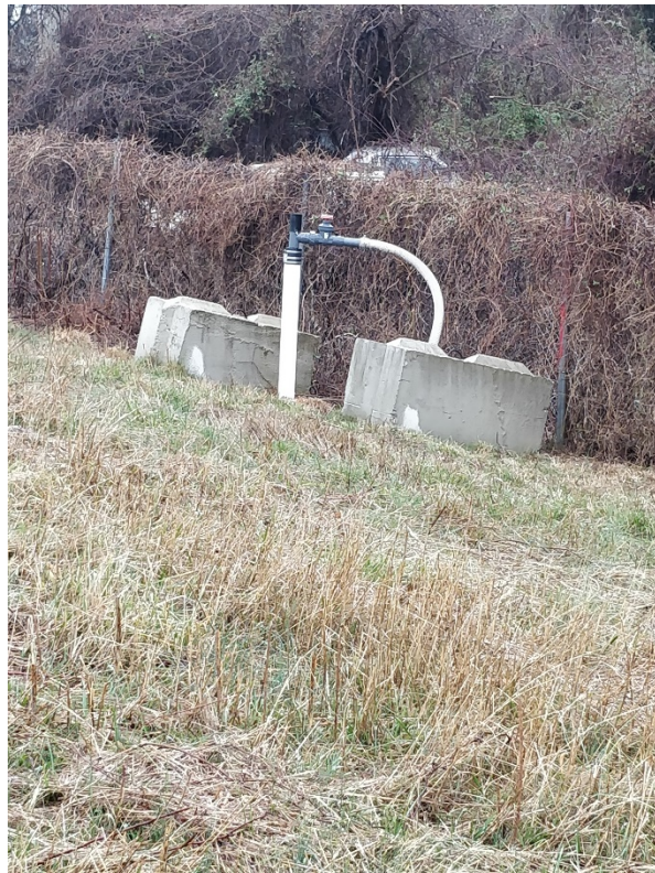
Landfill gas extraction well near the toe of Grantham South Area
