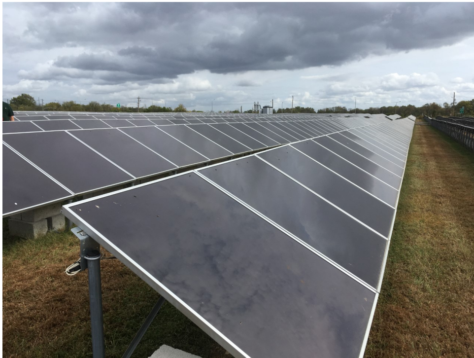
Solar array on South Landfill
