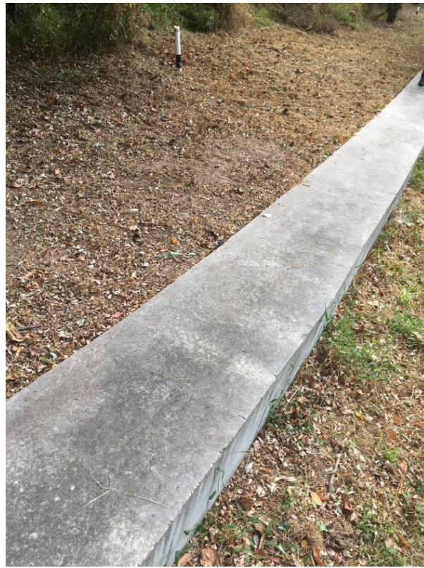
Cement knee wall at North Landfill with piezometer in background
