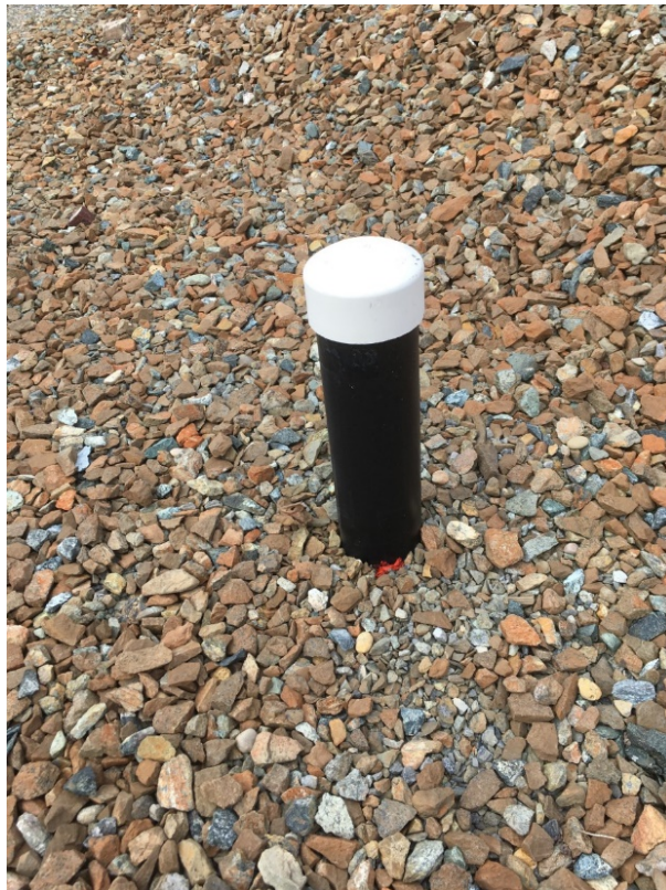
Extraction trench cleanout CL-3 in the BASF plant area
