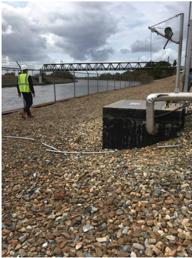
Extraction well EW-1 at BASF plant area
