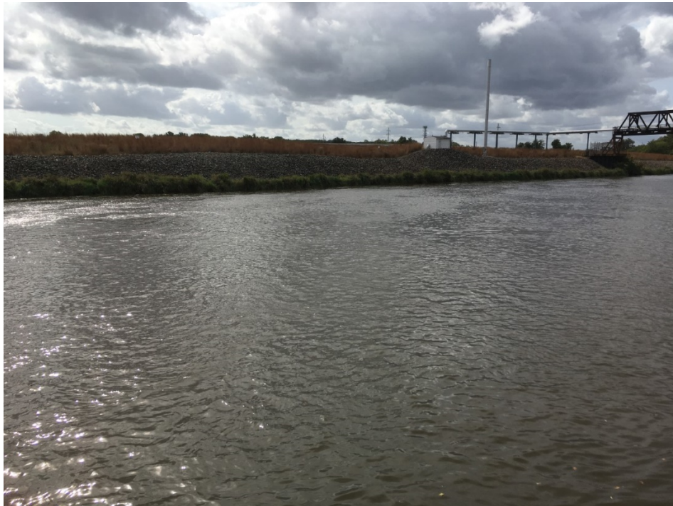
Christina River with South Landfill in the background
