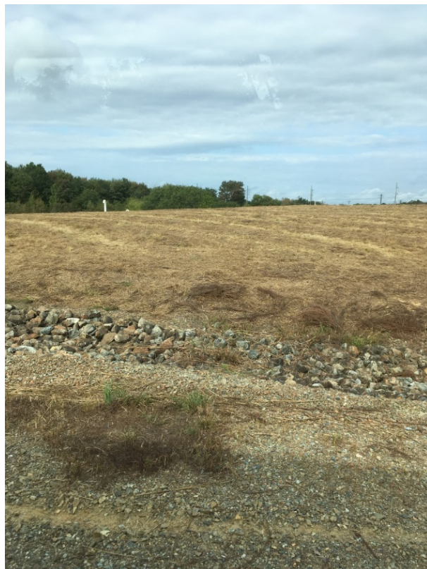
North Landfill with perimeter rip-rap lined drainage channel
