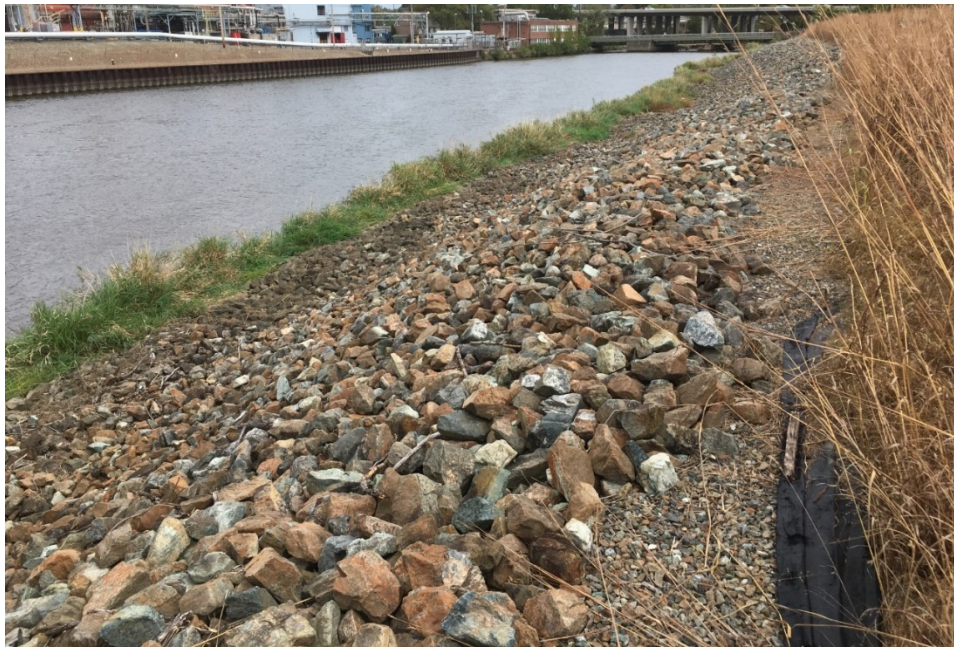
Stabilized bank along South Landfill
