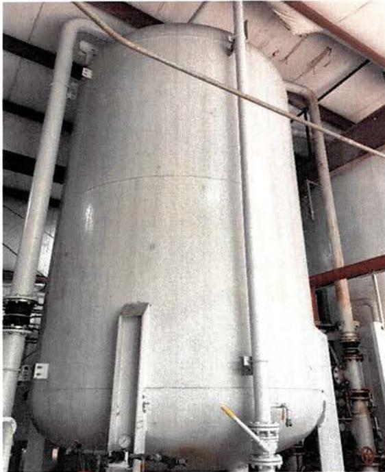
Picture 2. Granular activated carbon unit (20,000 pound)
