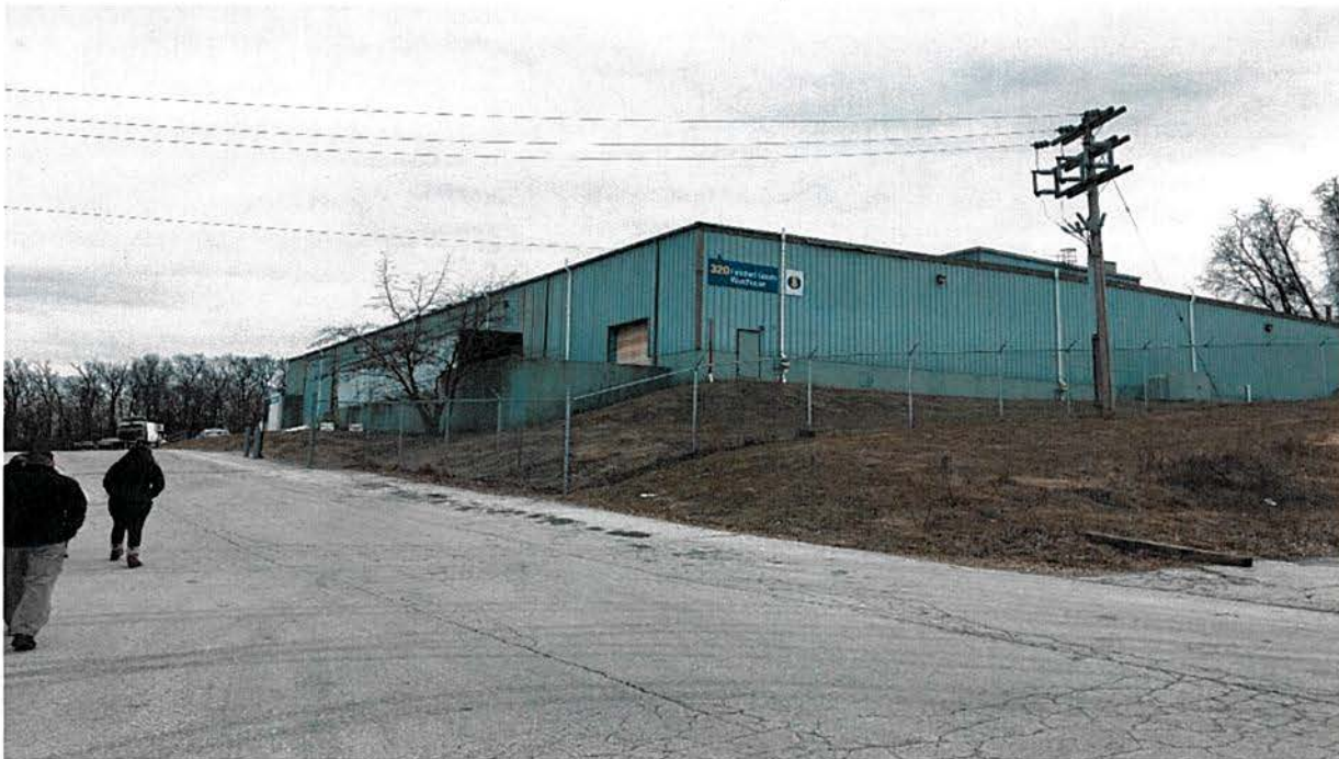
Picture 2. Warehouse with VI mitigation system.
