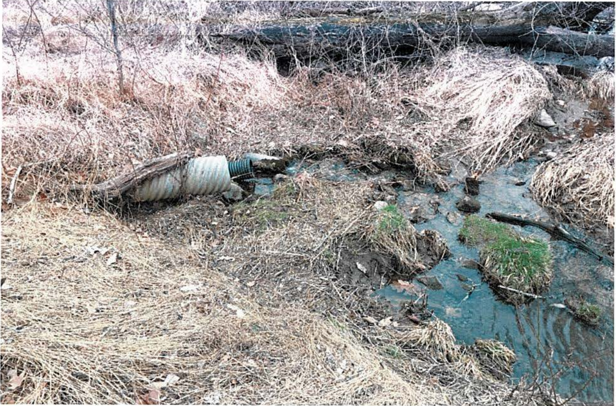
Picture 7. Treated groundwater outfall.
