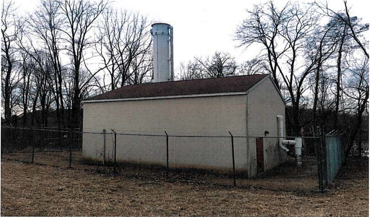
Picture 5. Groundwater treatment building.
