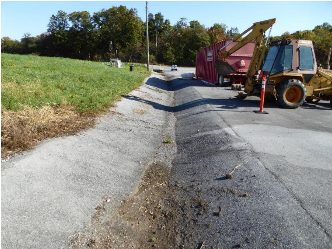
Surface water runoff collection ditch.
