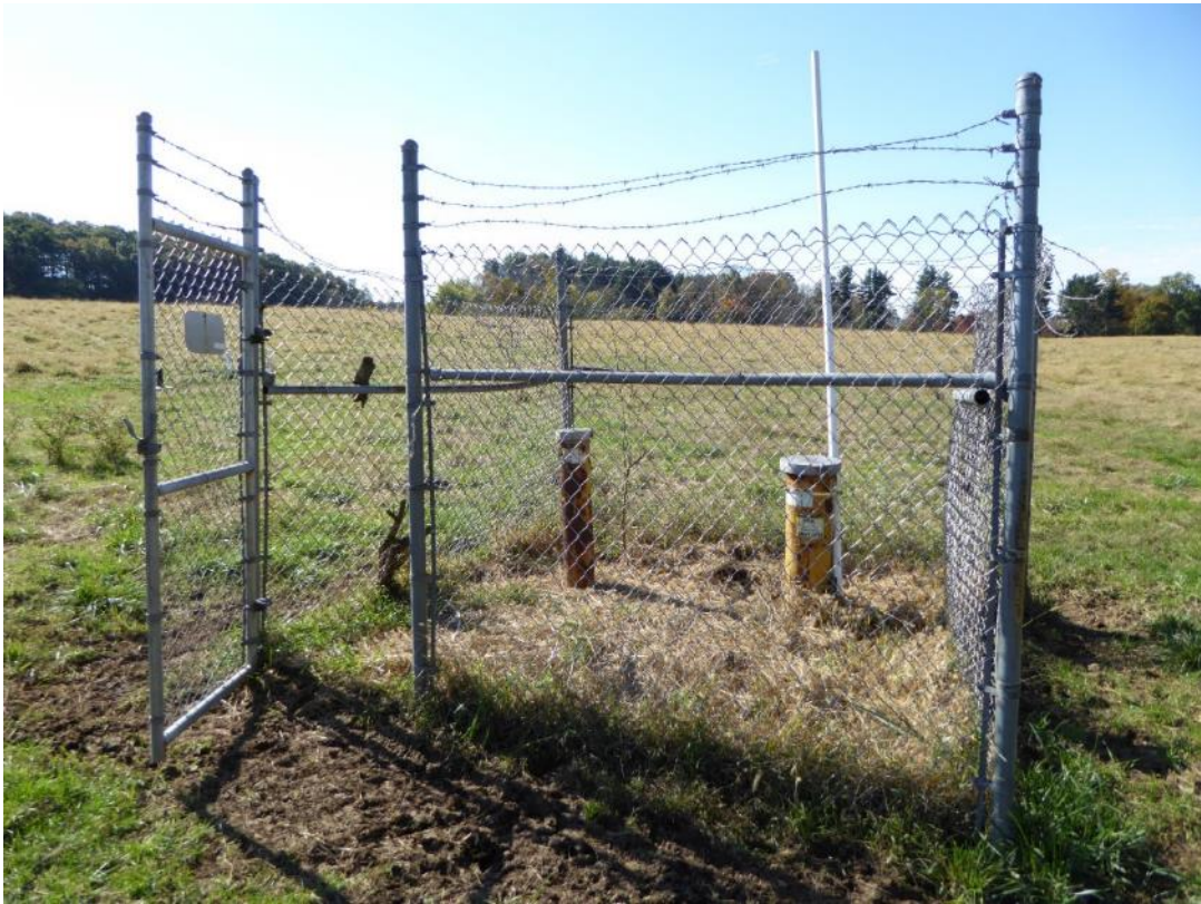
Monitoring well ED11IR in cow pasture. Gate is not locked.
