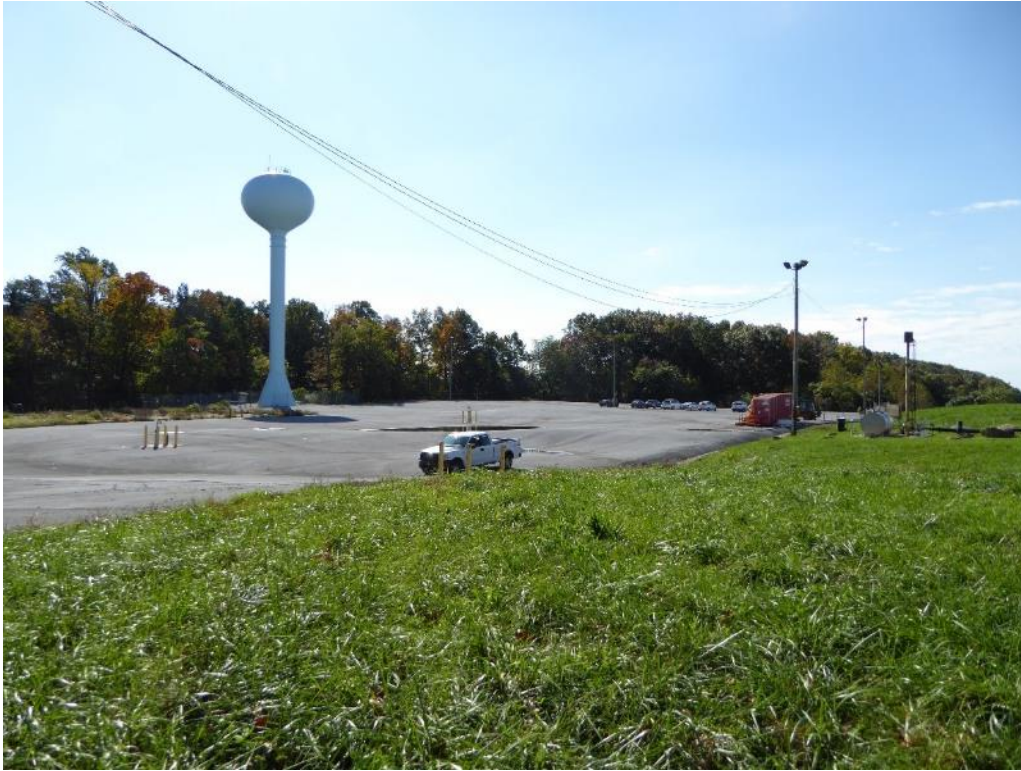
Asphalt cap and water tower on site property. Gas flare is at right.
