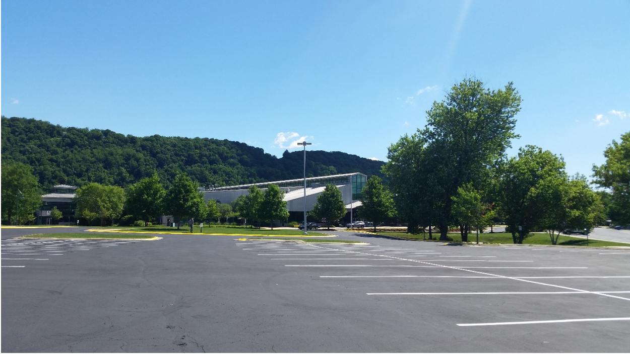
Figure 5 - Golf Dome Parking Lot (capped area)
