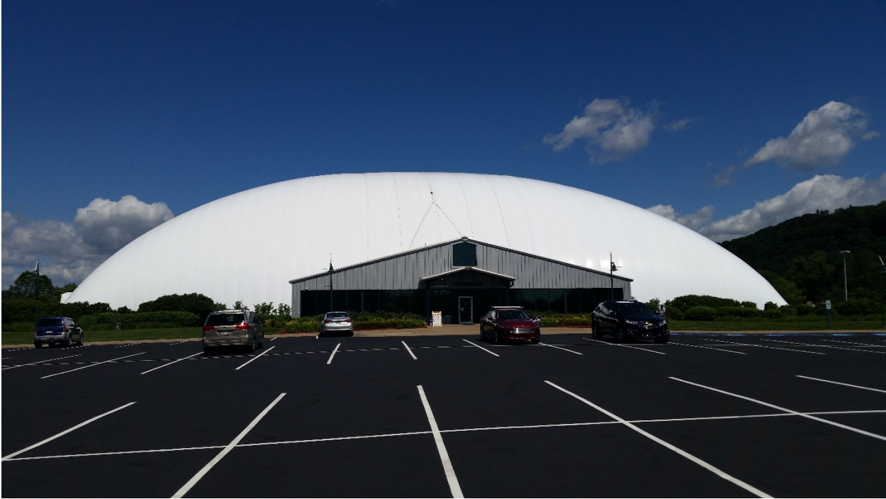
Figure 6 - Golf Dome (capped area)
