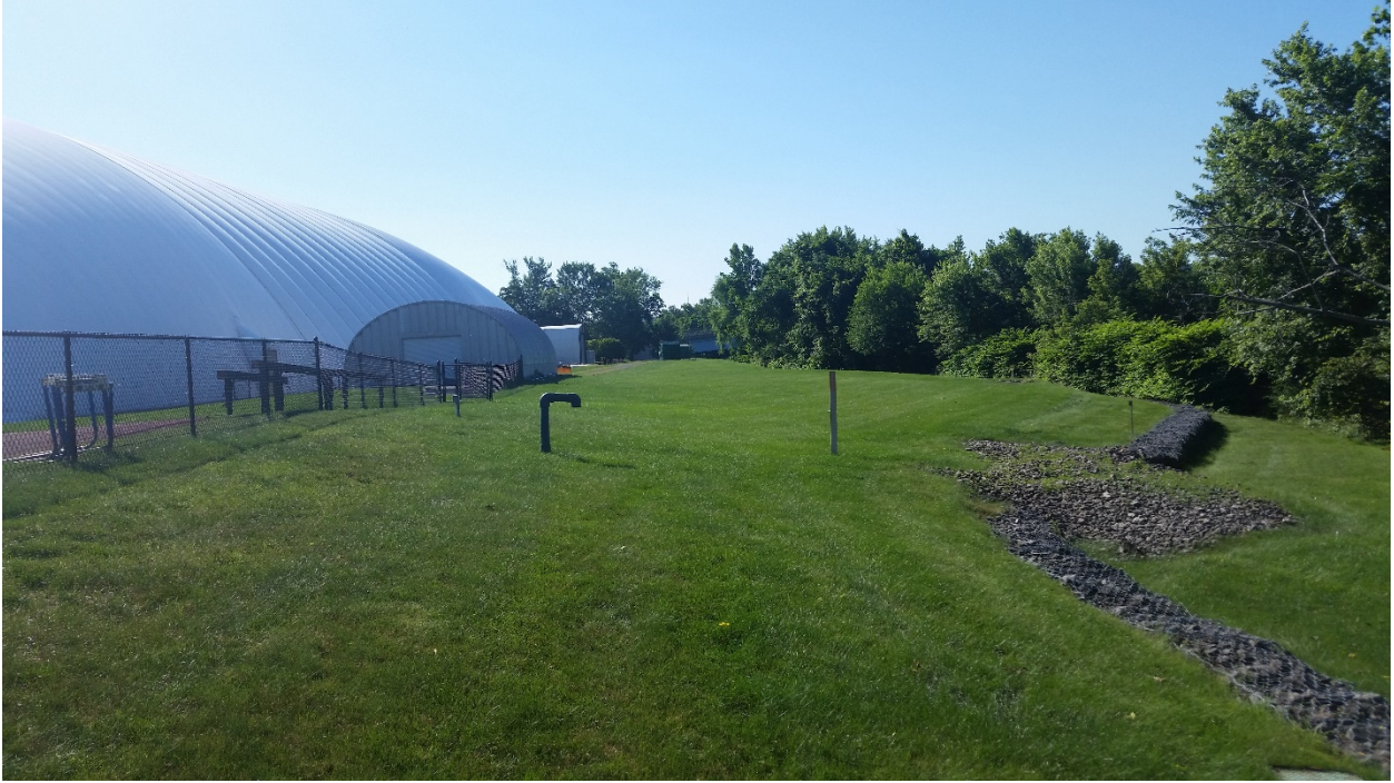
Figure 7 - Approximate Location of Slurry Wall
