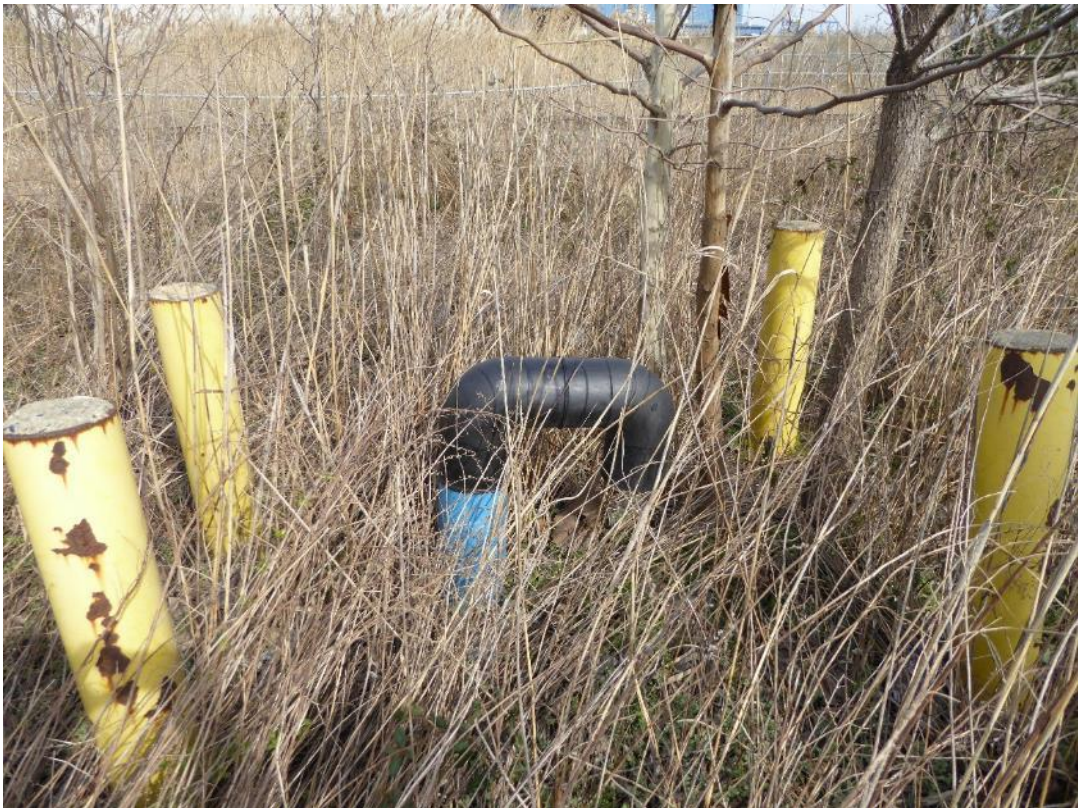
Passive gas vent at carbon disulfide treatment area
