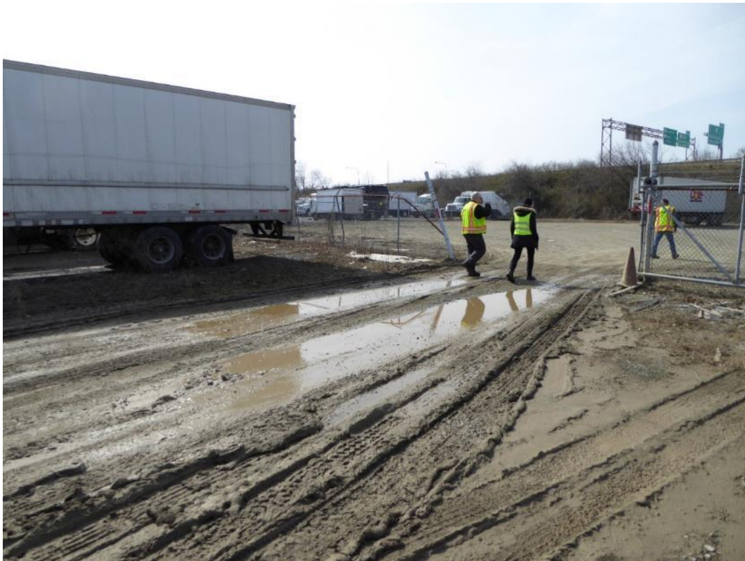
Ponding on aggregate cap at truck stop
