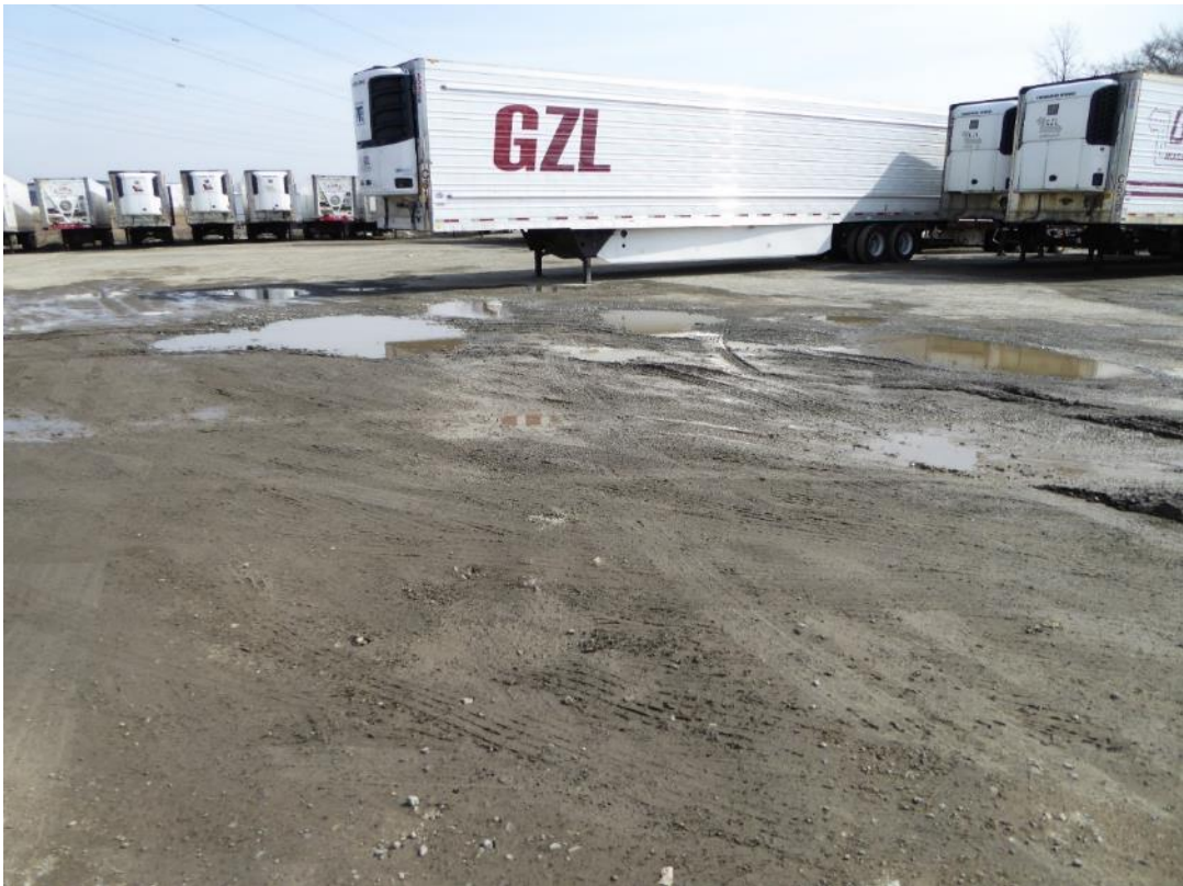
Ponding on aggregate cap at truck stop
