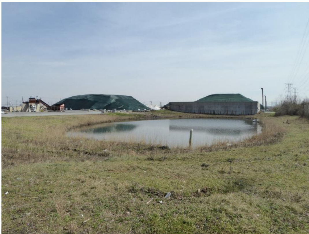
Pond at northwestern end of capped former marsh area on Potts Property. Background: concrete pad constructed on top of excavated drainage ditch sediments.
