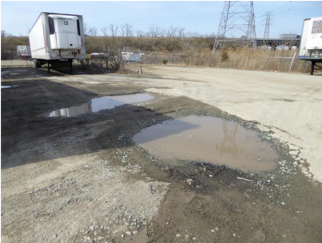
Ponding on aggregate cap at truck stop
