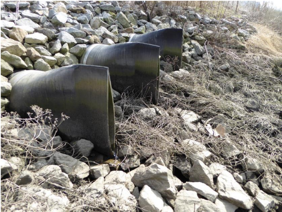
Outlet structure from Halby stormwater pond into I-495 ditch
