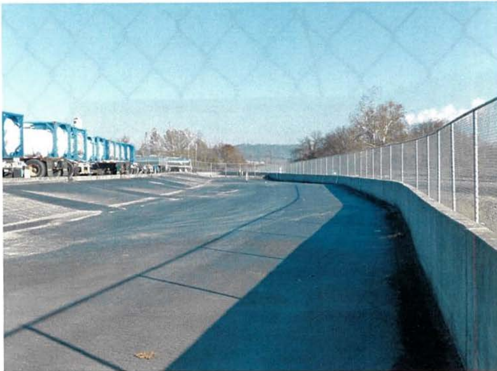
Stormwater management feature along the eastern edge of the Chemical Plant property cap.
