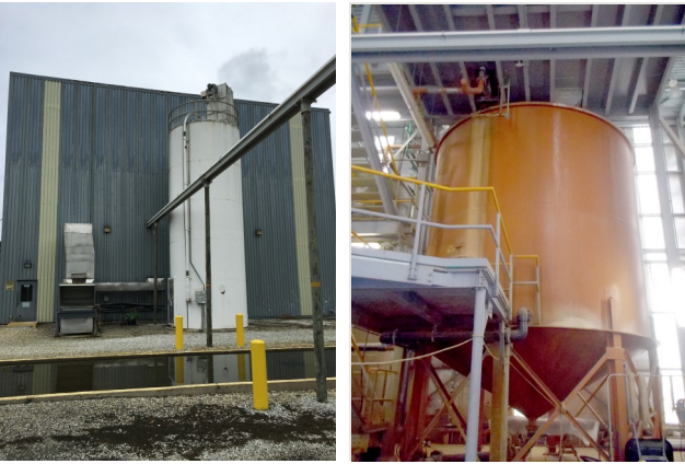
Bottom: Outdoor and indoor images of the on-site pump and treat system. This system, which has been operating since 1996, treats acidic groundwater, which is then discharged into the Piney River.
