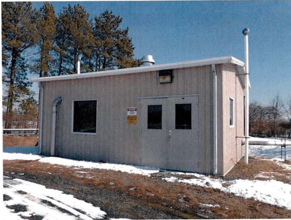
The blower building is located at the far northeast corner of the main landfill.
