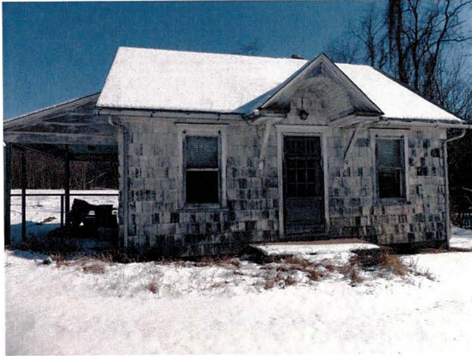
In 1976, groundwater contamination was first discovered at the Wagner well, located next to this abandoned house. This house is located on the Wagner property, east of the Site.
