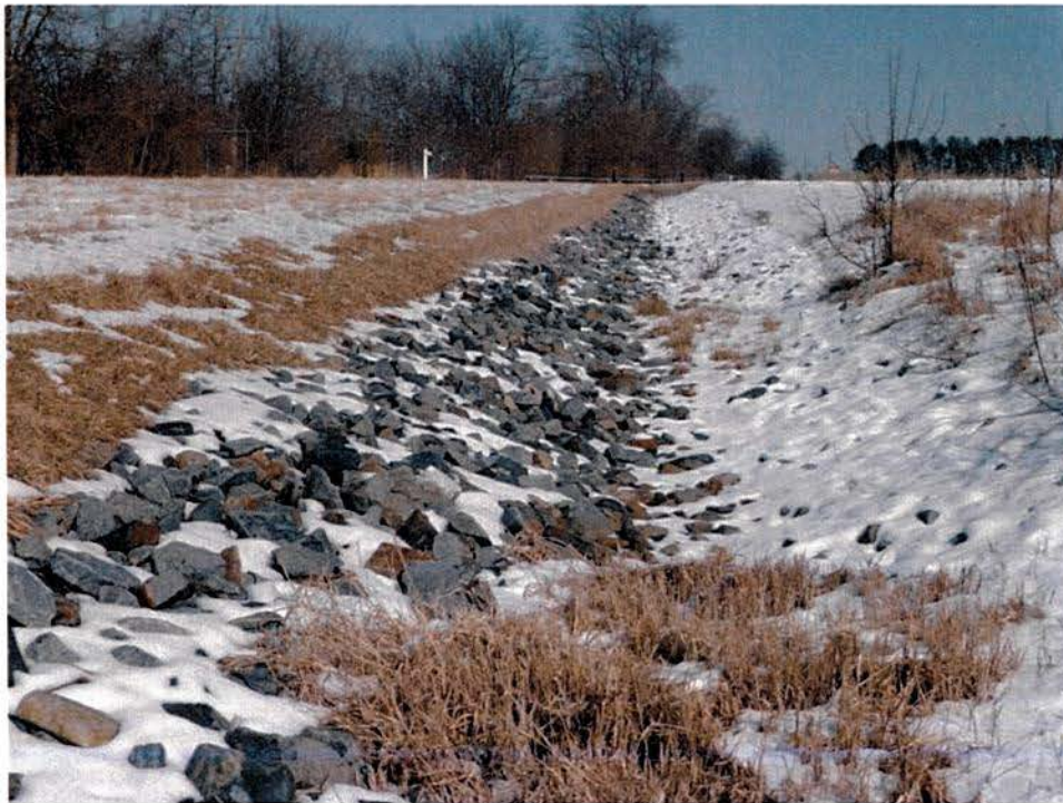
This perimeter drainage ditch surrounds the main landfill.
