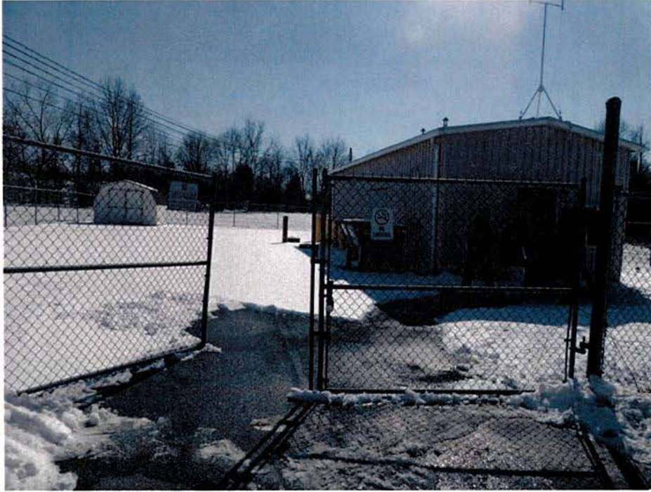
This locking gate on Site restricts access to the pump house.
