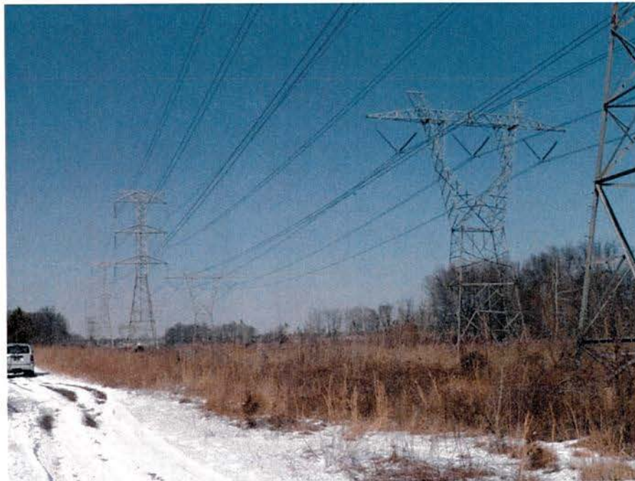
The Delmarva Power & Light Co. has a right-of-way across the southwestern part of the Site. The power lines run between the main landfill and west fill areas.
