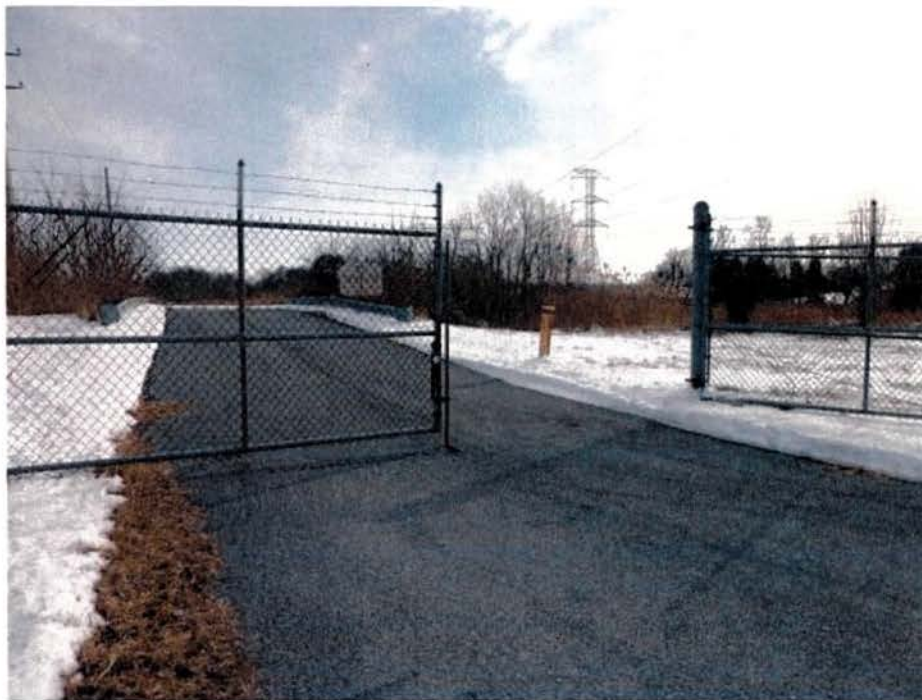
This locking gate secures the Site entrance.
