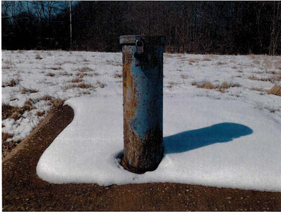
On-site groundwater monitoring well TY-208 was locked at the time of the Site inspection.
