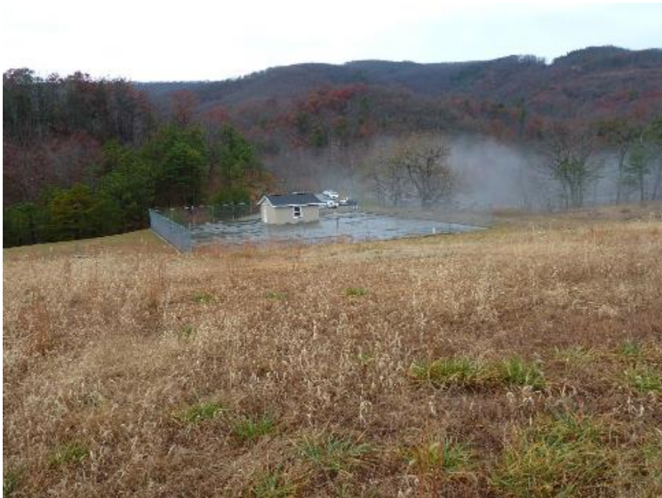
Looking west from monofill to police training building
