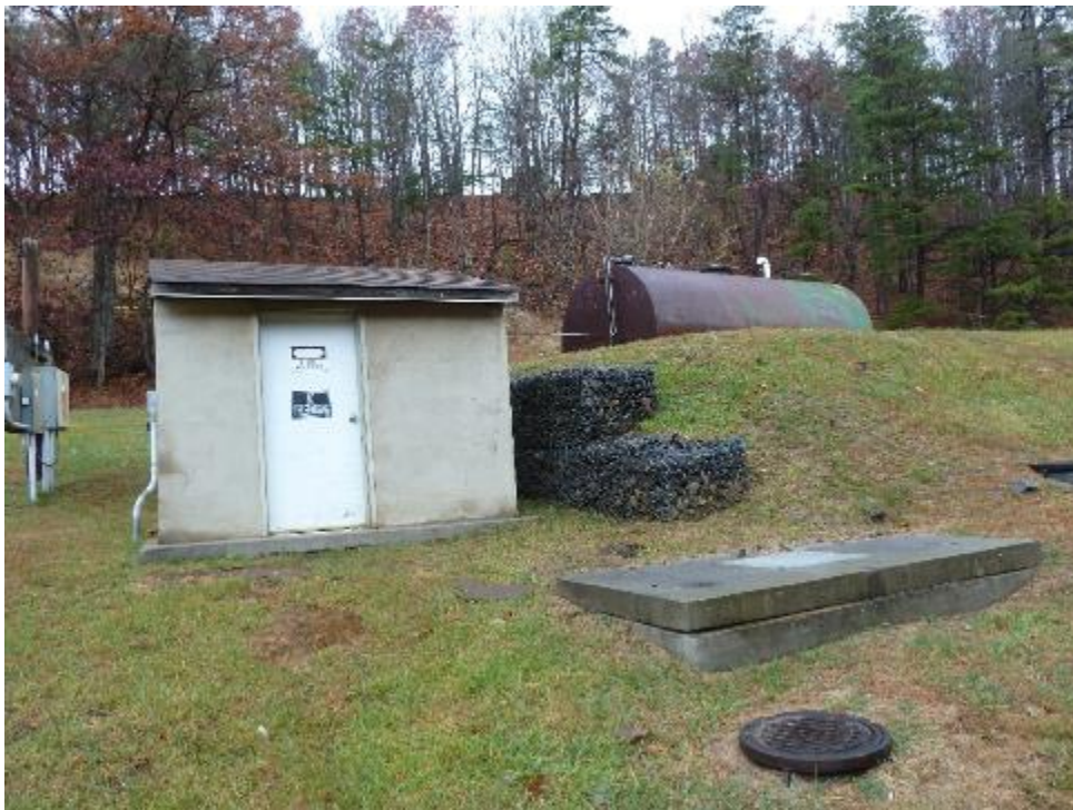
Inactive leachate collection tank, municipal water supply pump house and leachate vault
