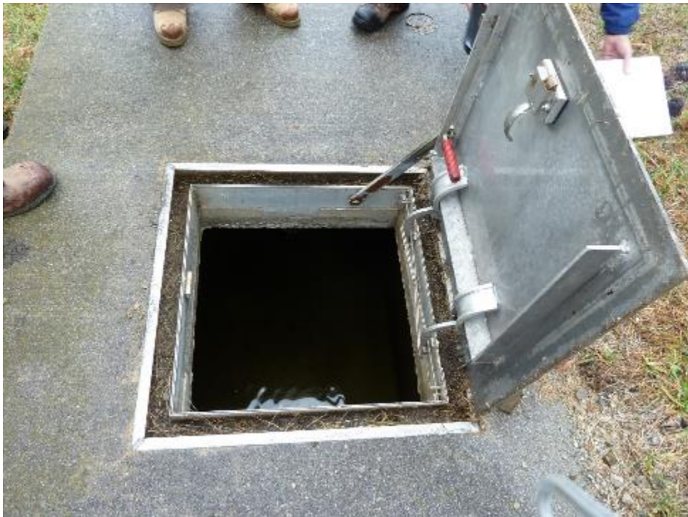
Looking into leachate vault
