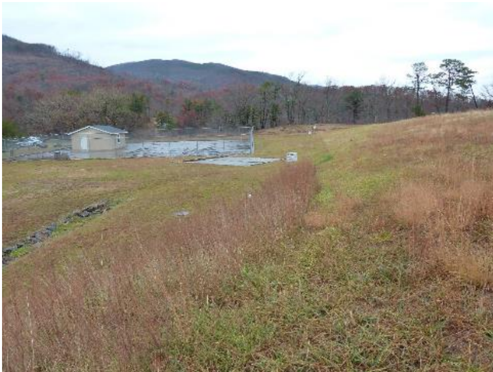
Looking north from eastern side of monofill to police training building
