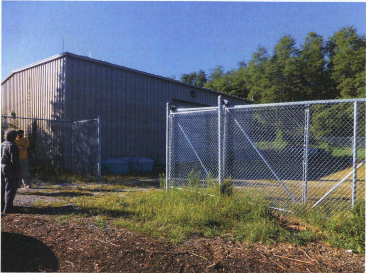
Entry to treatment building.
