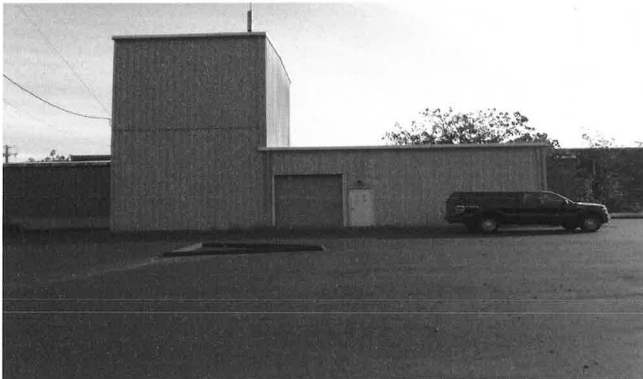
Hellertown Manufacturing Co. Superfund Site – Fourth Five-Year Review Groundwater Treatment Plant Building Looking West across the Paved (Former Lagoons) Area.
