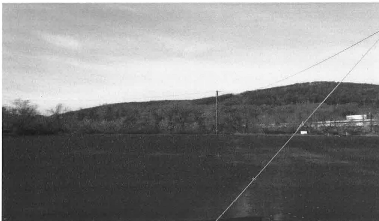
Hellertown Manufacturing Co. Superfund Site – Fourth Five-Year Review Former Lagoon Area Looking East from the Groundwater Treatment Plant Building
