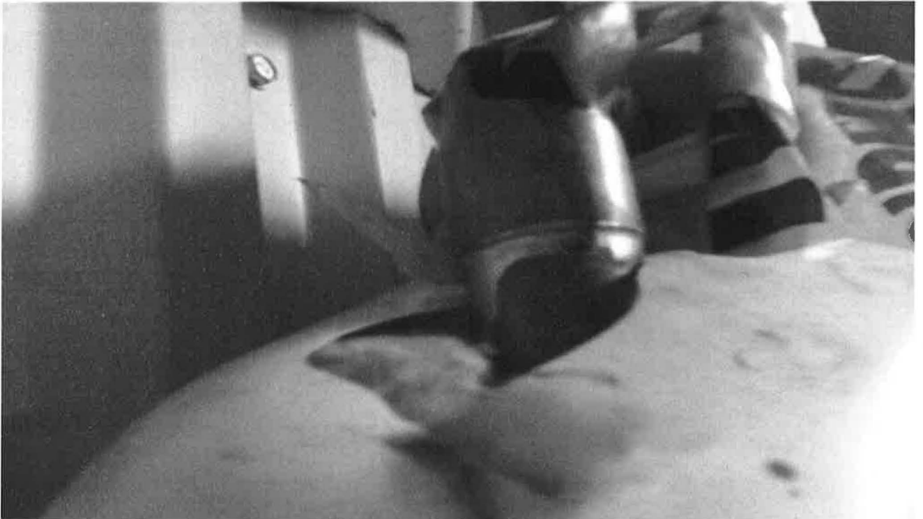
Hellertown Manufacturing Co. Superfund Site - Fourth Five-Year Review Freeze/Thaw Damage to Treatment Plant Piping
