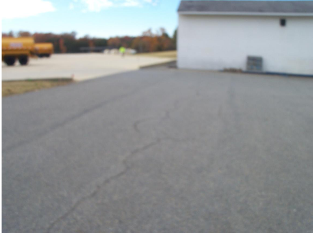
Minor crack on asphalt cover.
