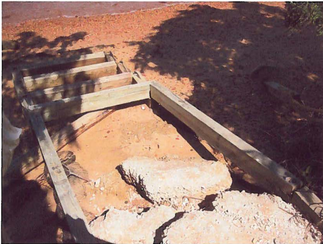
Photo 3 Storm damage to beach access timber stairs Between swales AA and BB, Site 1
