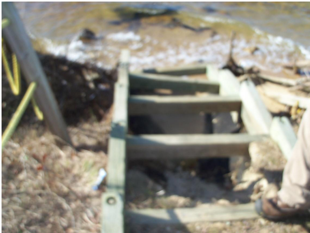
Erosion beneath stairway at Site 1 boundary observed during 11-16-12 inspection.
