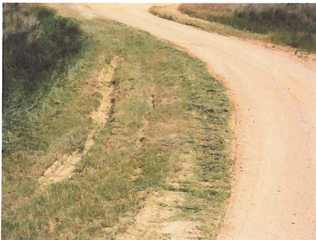
Photo 2 Tire rut off west edge of central access road Site 1
