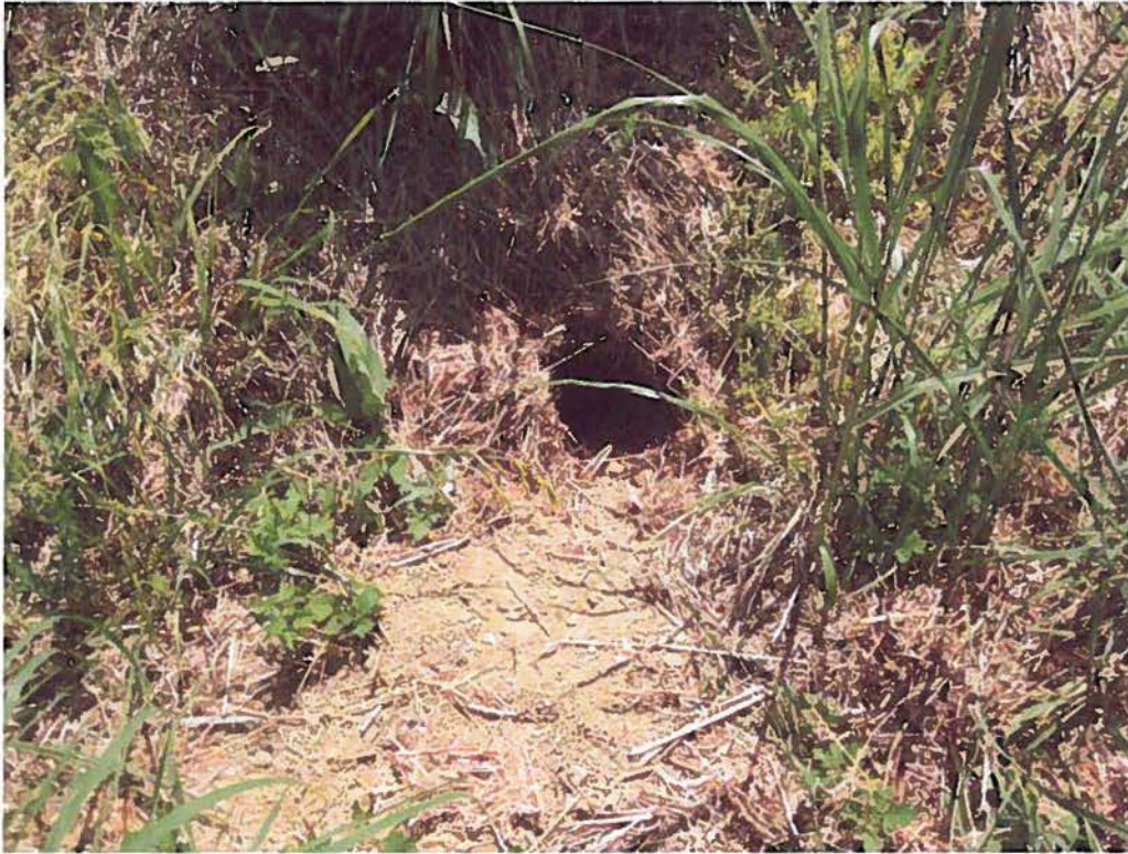
Photo 1 Inactive rodent hole on Northwest landfill slope (filled subsequent to inspection date)
