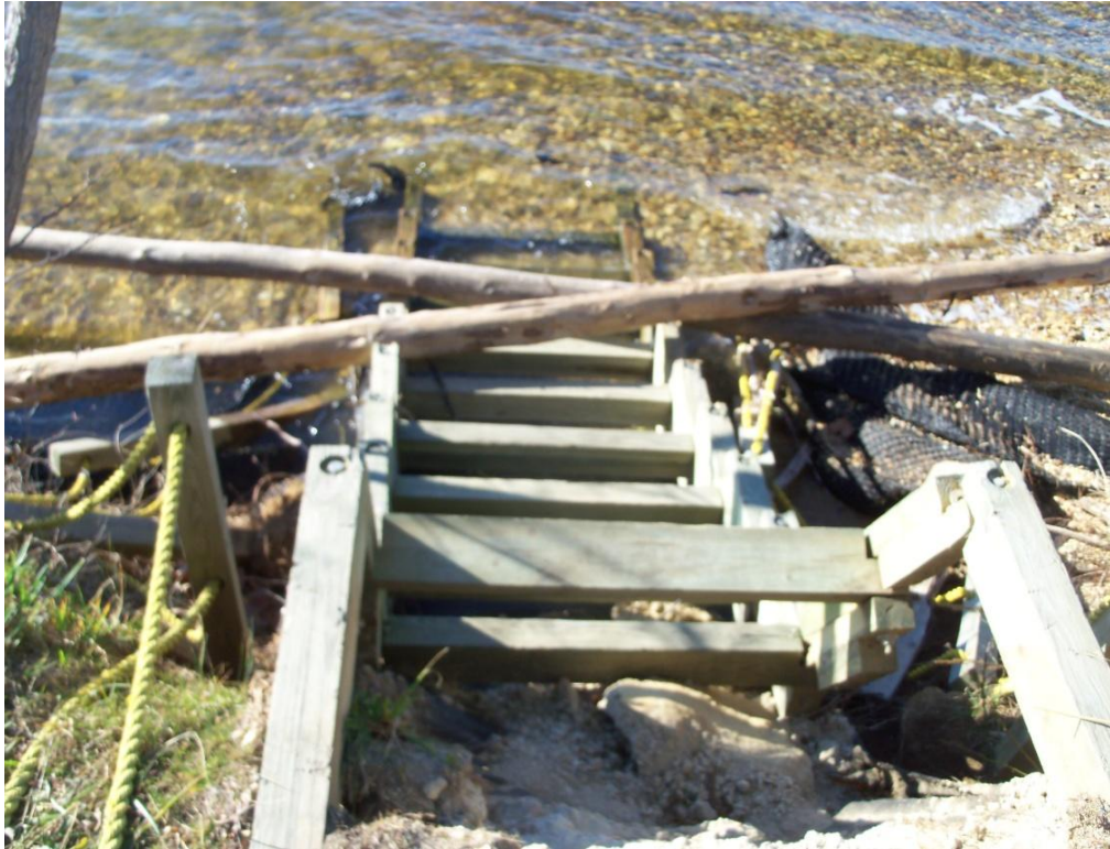
Erosion beneath stairway at Site 1 boundary observed during 11-16-12 inspection.
