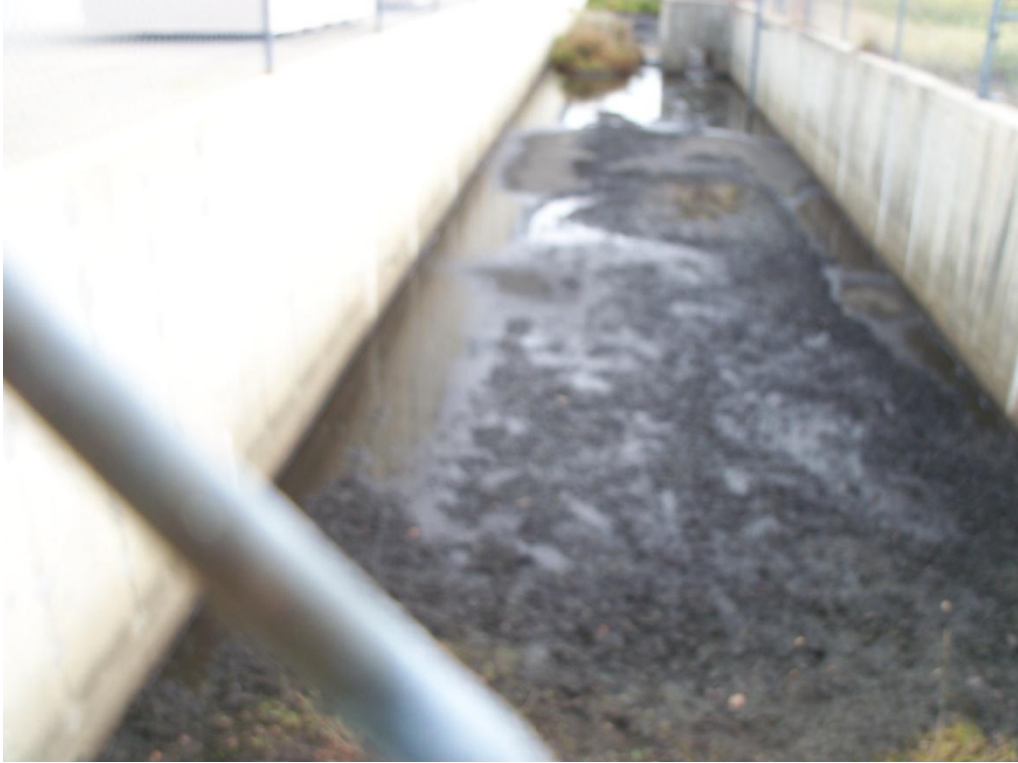
Minor sedimentation in containment area.
