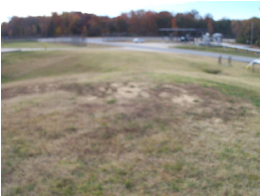
Very minor erosion on soil cover along western site boundary.
