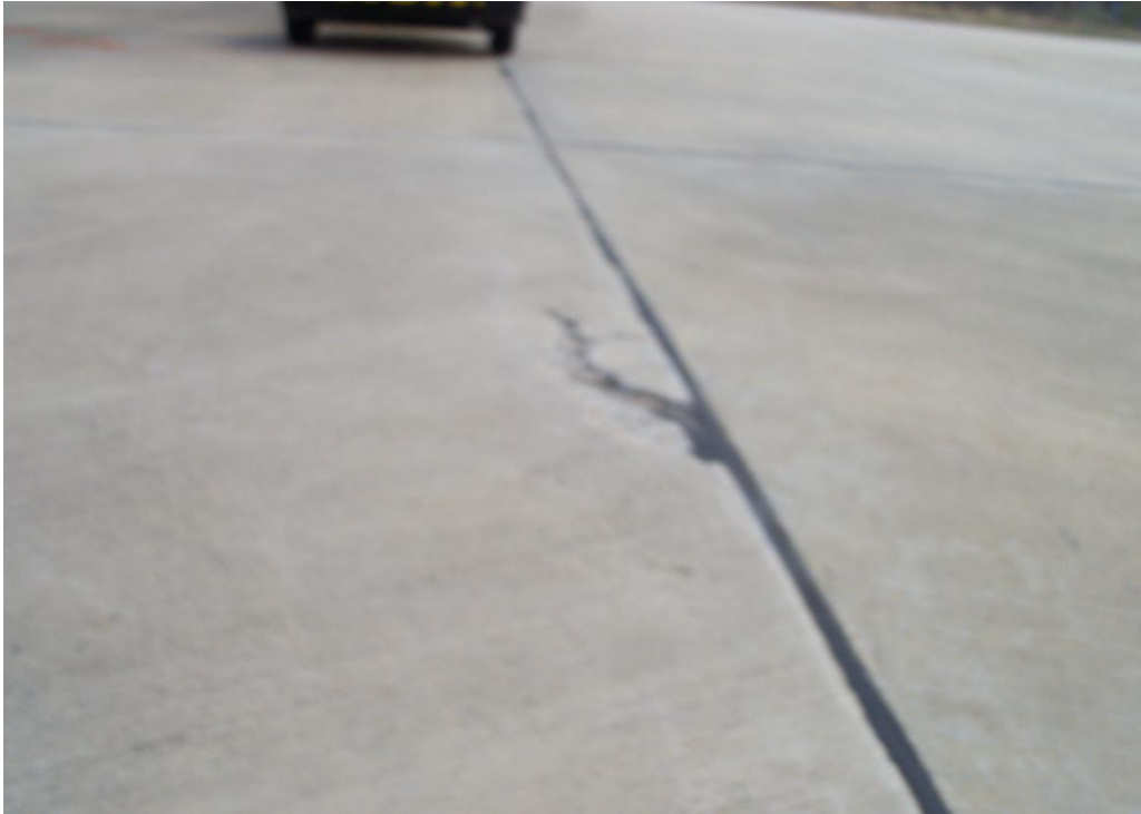
Very minor crack on concrete cover.
