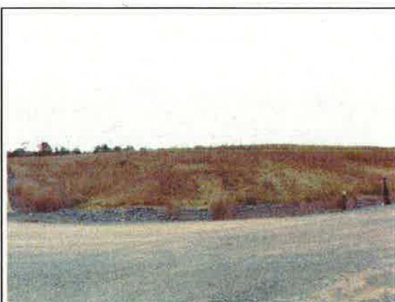
Photo 8: Viscous Basin 2 & 3 (10-23-12) Latitude: 38.9297 Longitude: -78.21408 Description: Unstable soils with sparse to bare vegetation
