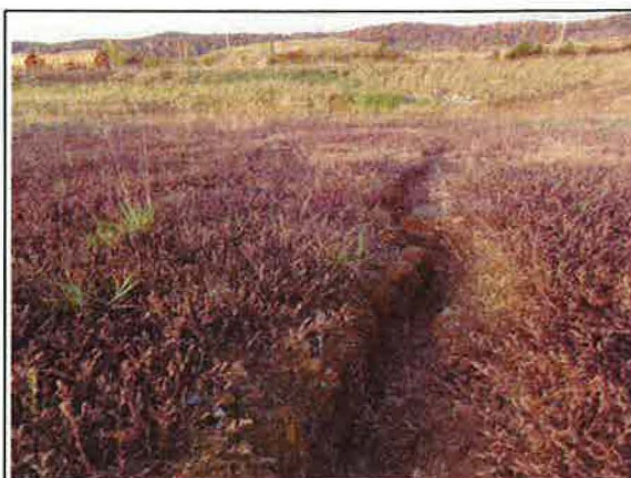
Photo 4: Storm Water Basin East (10-23-12) Latitude: 38.9221 Longitude: -78.21543 Description: Erosion Gullies North of Basin
