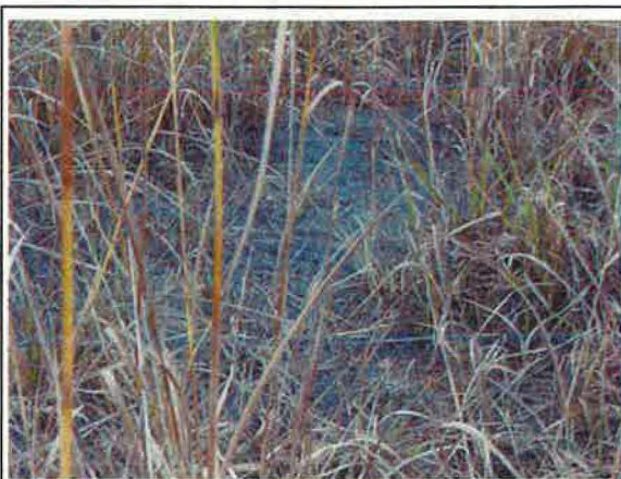
Photo 18: FAB-6 (10-23-12) Latitude: 38.91957 Longitude: -78.21115 Description: Sparse vegetation & exposed TRM matting along ditch
