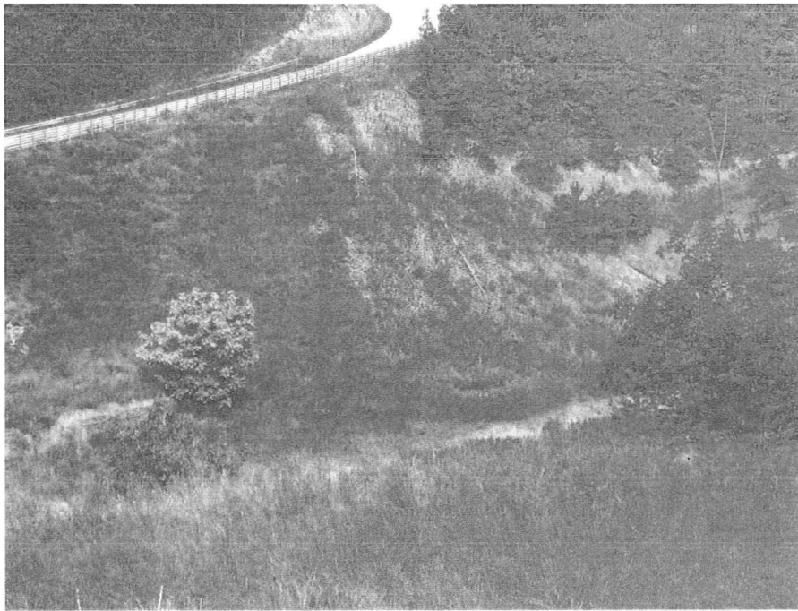
Photo 9. The ravine with the culverted stream.
