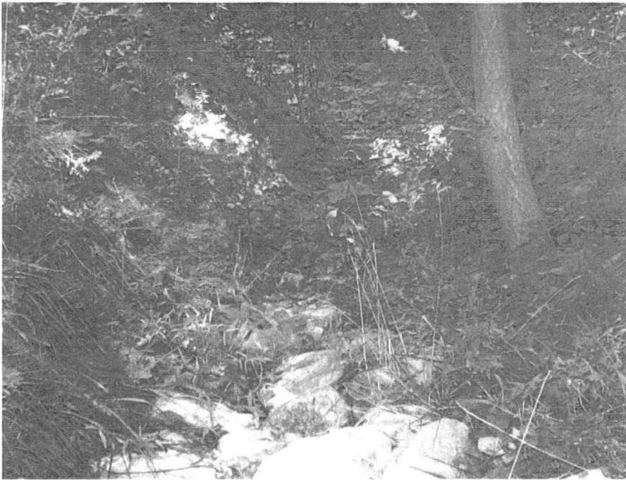
Photo 13. The start of the stream from the culvert. The stream is dry in this photograph.
