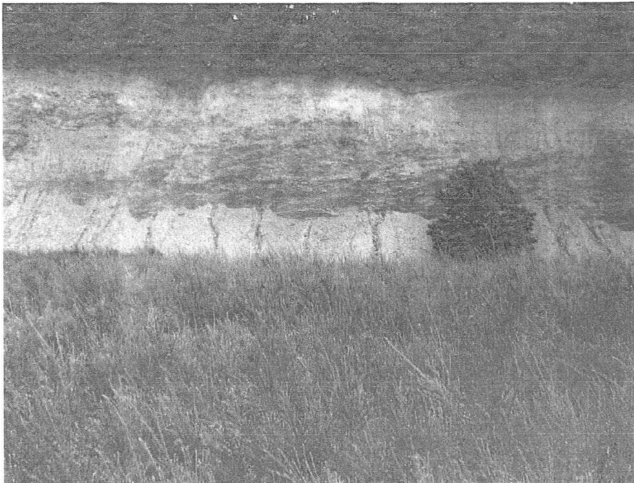
Photo 5. A view of the monofill cap and the hillside east of the cap.
