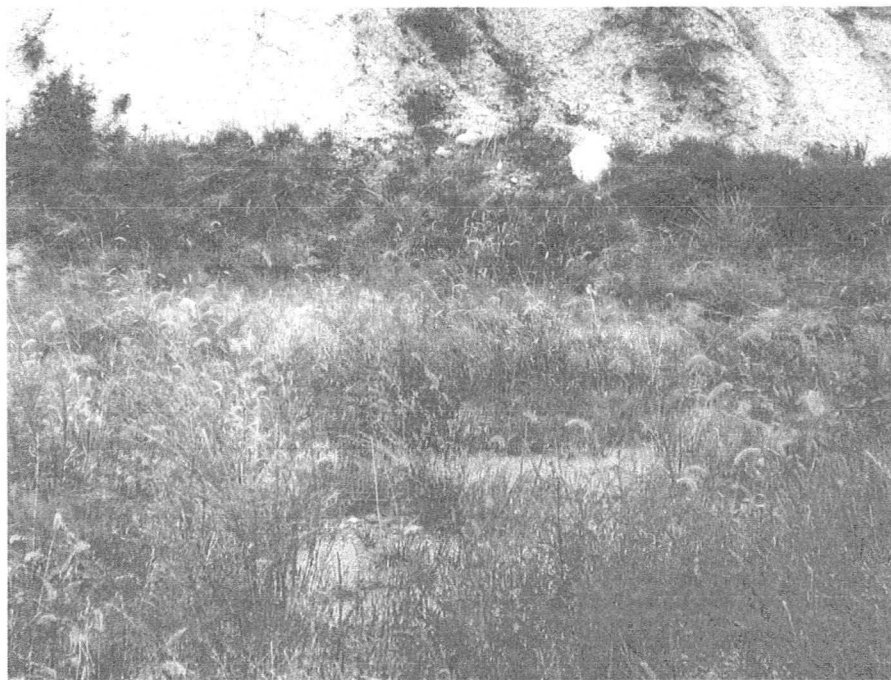
Photo 6. On the east side of the monofill cap there appears to be a depression with sparse vegetation.
