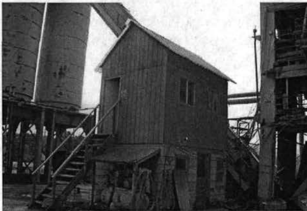
Control House II, Looking Southwest (Photo taken by Paul Griffith on August 8, 2011)
