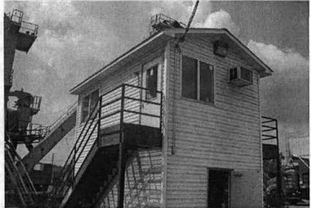
Control House, Looking Northwest (Photo taken by Paul Griffith on August 8, 2011)
