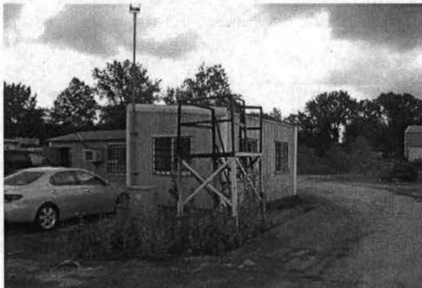
Laboratory Building, Looking East (Photo taken by Paul Griffith on August 8, 2011)
