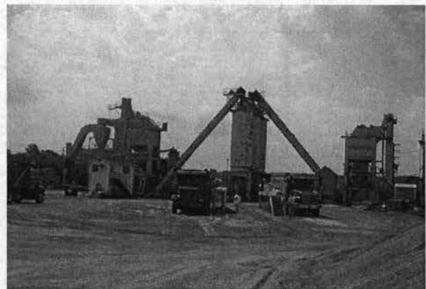
Asphalt Plant, Looking South
