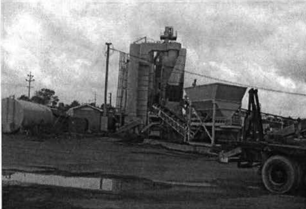
Asphalt Plant Equipment, Looking West (Photo taken by Paul Griffith on August 8, 2011)
