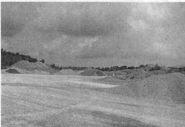
Material Area, Looking North
