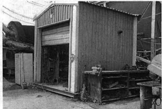
Power Building, Looking Northwest (Photo taken by Paul Griffith on August 8, 2011)
