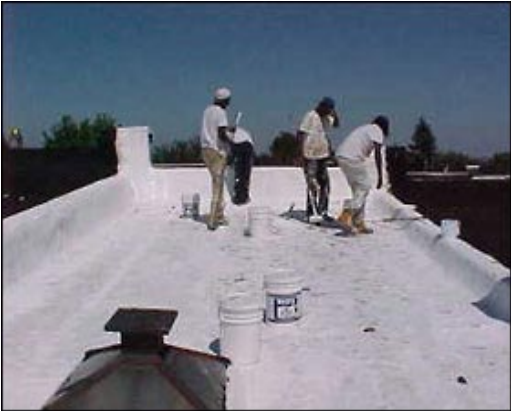
Figure 9: Reflective roofing material being applied to a rowhouse in Baltimore
