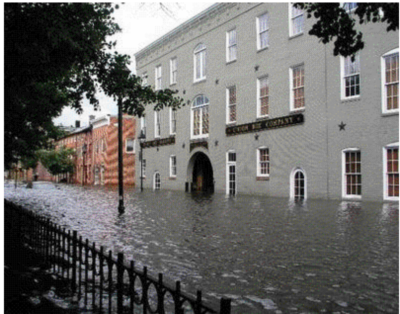
Figure 3: Lancaster Street, Fells Point after Hurricane Isabel, 2003
