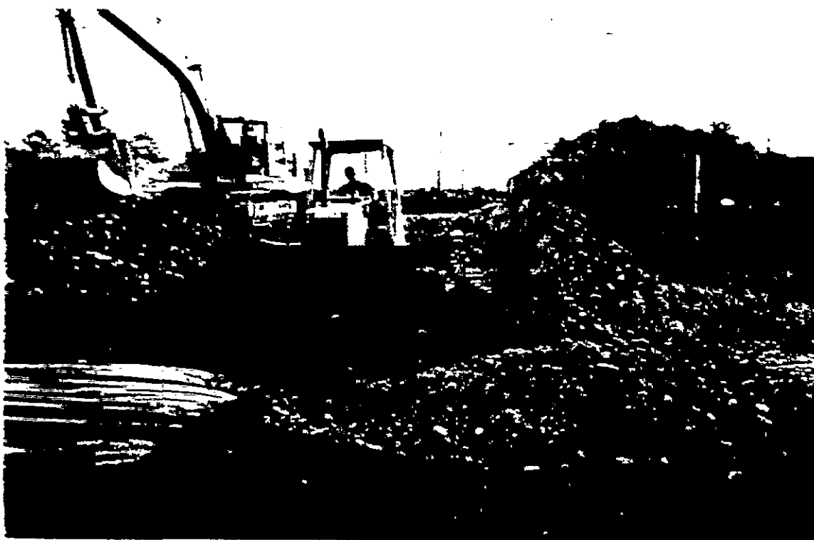
Photo 7: Soil anchor being placed on sides of Test Pad 3 (Sulfate Basin 3).
