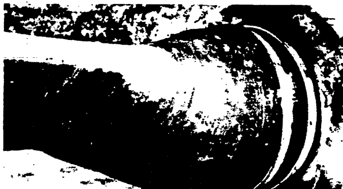
New York's 54" Tide-Flex as interceptor discharge valve.
