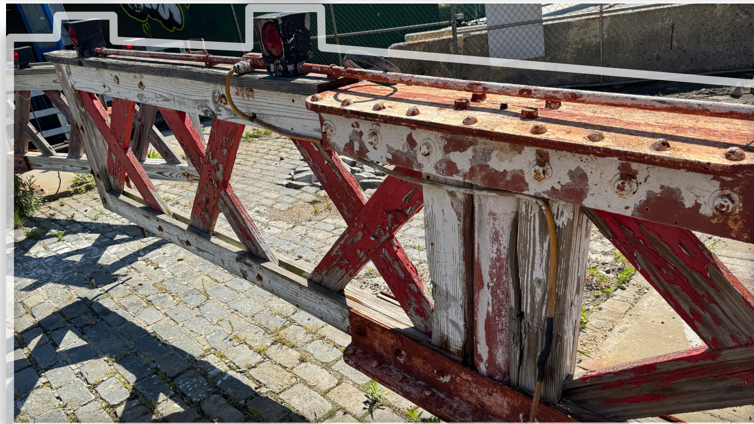
② EAST ABUTMENT VIEW LOOKING EAST PHOTO OF EXISTING BARRIER GATE
