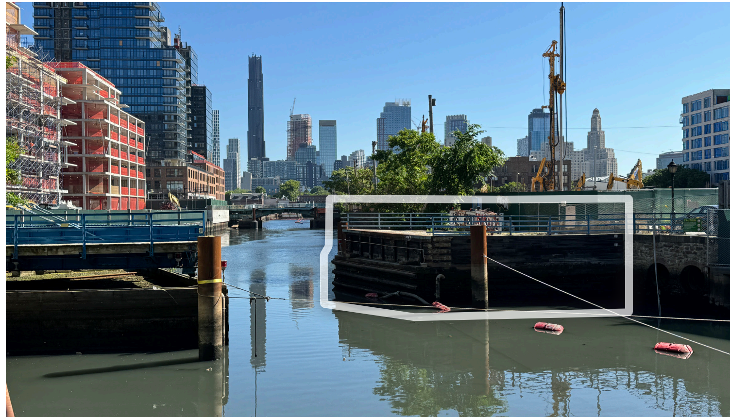
① CARROLL ST BRIDGE VIEW LOOKING NORTHEAST PHOTO OF BRIDGE SOUTH ELEVATION FROM GOWANUS CANAL
