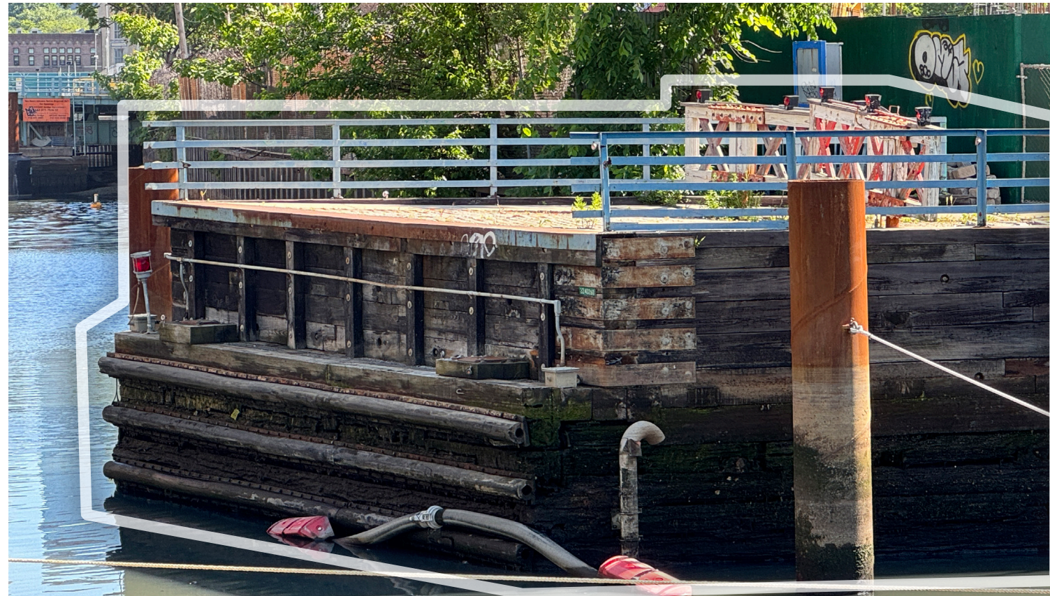
① EAST ABUTMENT VIEW LOOKING EAST PHOTO OF EXISTING TIMBER BULKHEAD
