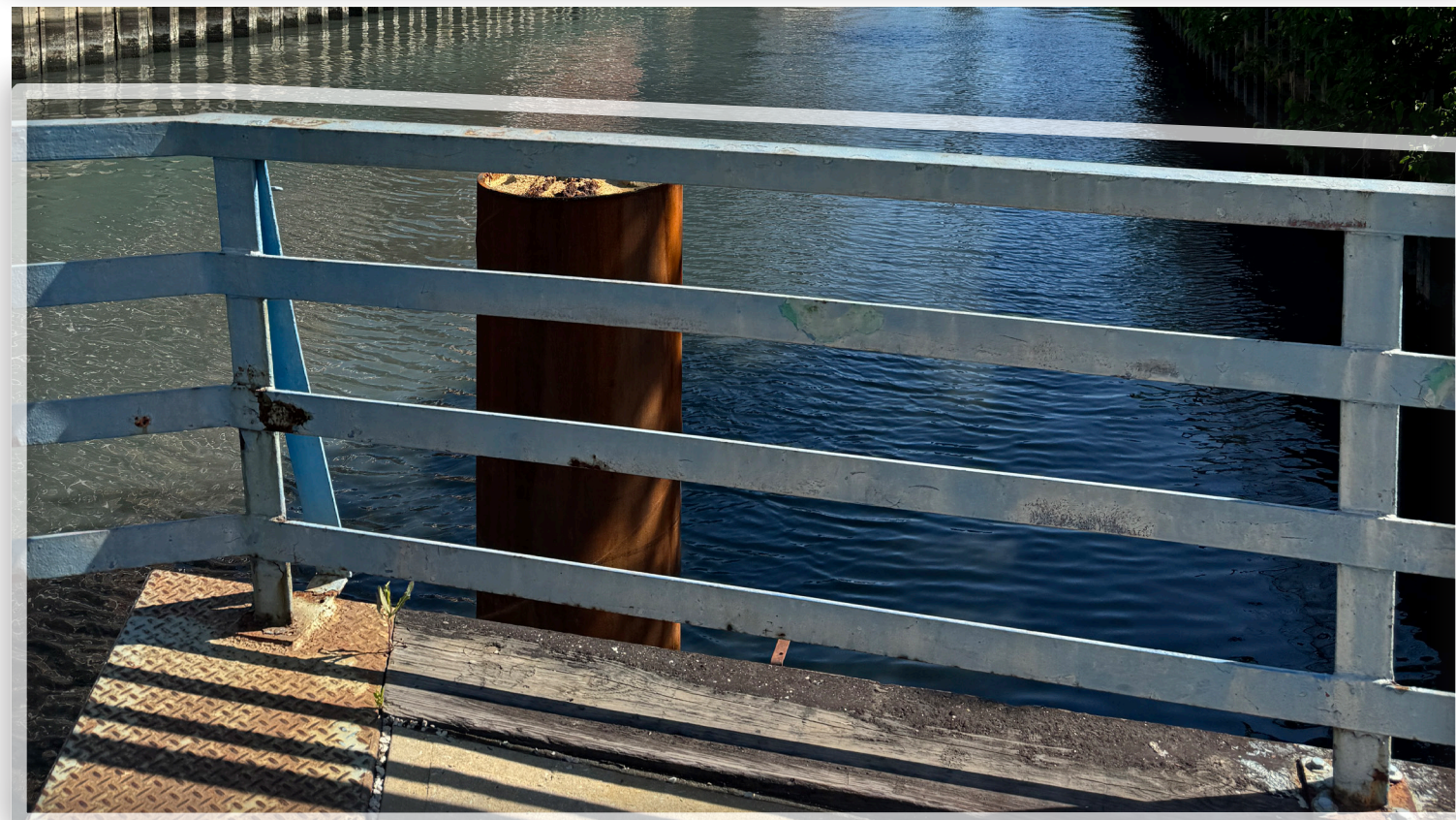
② EAST ABUTMENT VIEW LOOKING NORTH PHOTO OF EXISTING RAILING
