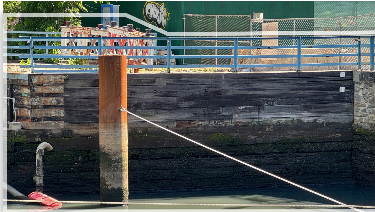
① EAST ABUTMENT VIEW LOOKING NORTHEAST PHOTO OF EXISTING TIMBER CRIBBING
