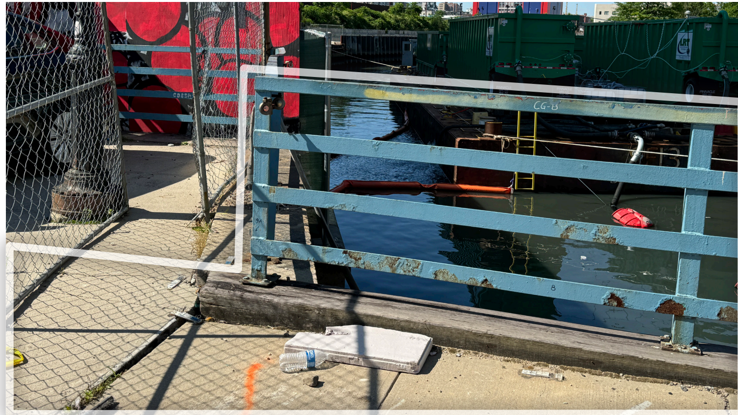
① EAST ABUTMENT VIEW LOOKING SOUTH PHOTO OF EXISTING SOUTH SIDEWALK, RAILING, AND CURB
