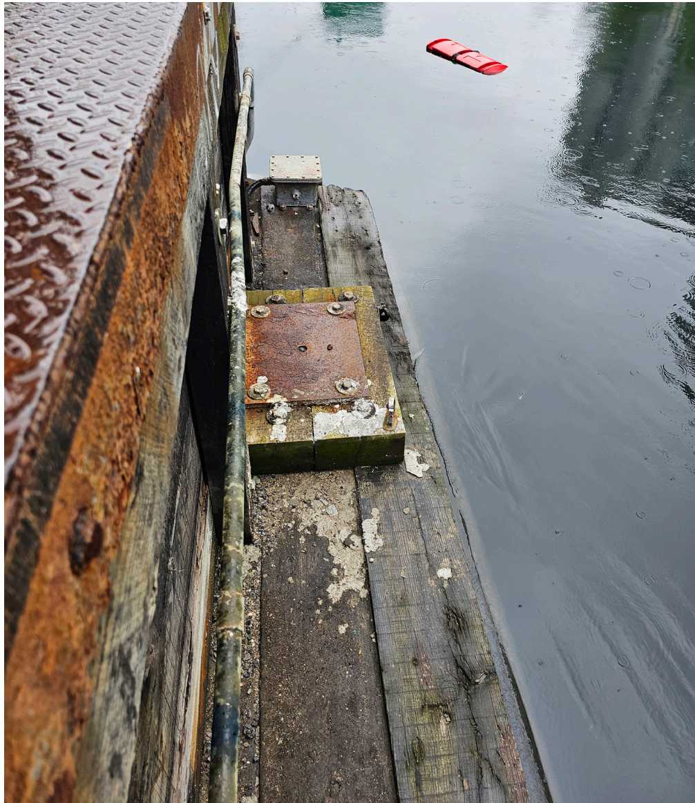
① SOUTH BRIDGE SEAT VIEW AT EAST ABUTMENT PHOTO OF CRIBBING SETTLEMENT TAKEN AT BRIDGE SEAT
