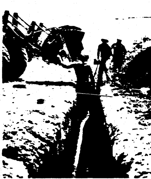
5 Backfilling trench with gravel for optimum support of pipe sidewall.
