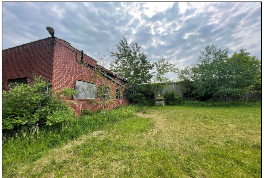
Part of the old American Thermostat Co. building at the site
