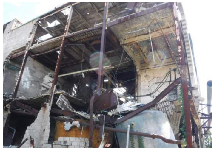
Exiting on-site structure slated for demolition
