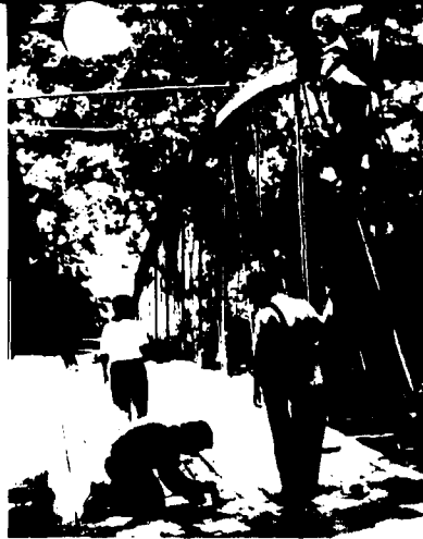
HAER technicians Lola Bennett, Robert Arzola, Sean O'Reilly, and J. Finbarr Garvey hand-measure the 116-year-old metal-truss Springfield-Des Arch Bridge, which survives near Springfield, Arkansas, largely due to its rural location (photo by Corinne Smith.)
