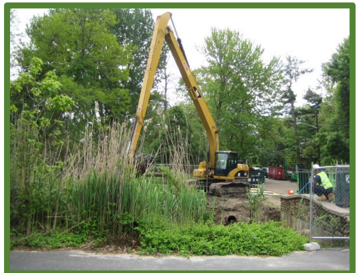
EPA removing PCB and lead contaminated soil
