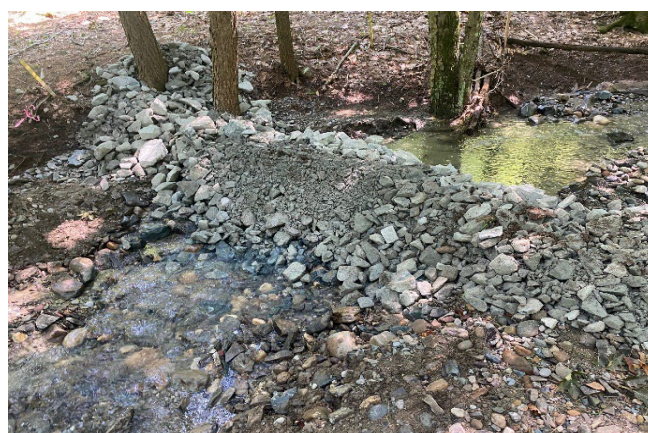
Stone dams installed near the outlet of Little Thunder Brook to reduce the downstream transport of sediment
