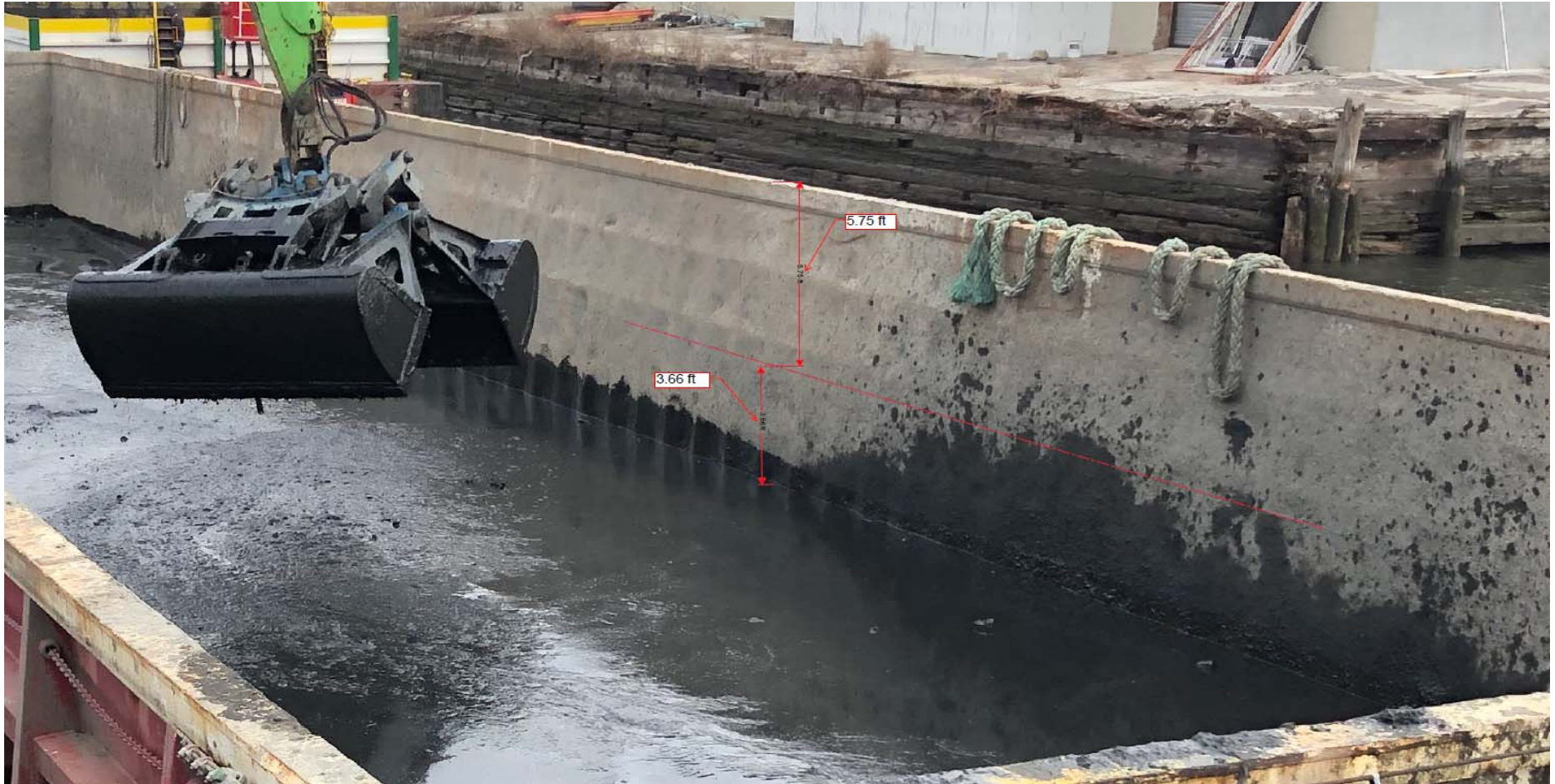
Photograph collected on Friday, January 22, 2021 prior to the Weeks #71 barge being transported to the Bay Ridge Flats mooring location. Distance from the weld line to the top of sediment is estimated as 3.66 ft.
