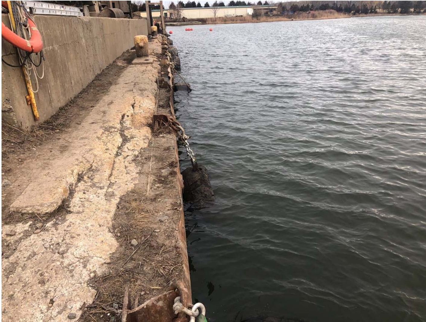
Photograph of newly installed tires serving as fenders at the docking location of the sediment processing facility. The tires protect the barge from metal shackles and H-piles along the bulkhead.
