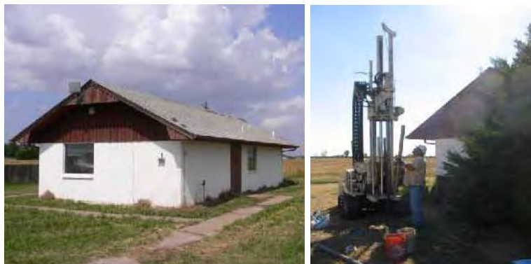
Geosyntec's industry-leading data quality assurance and control allowed us to clearly demonstrate the absence of vapor intrusion risks.
