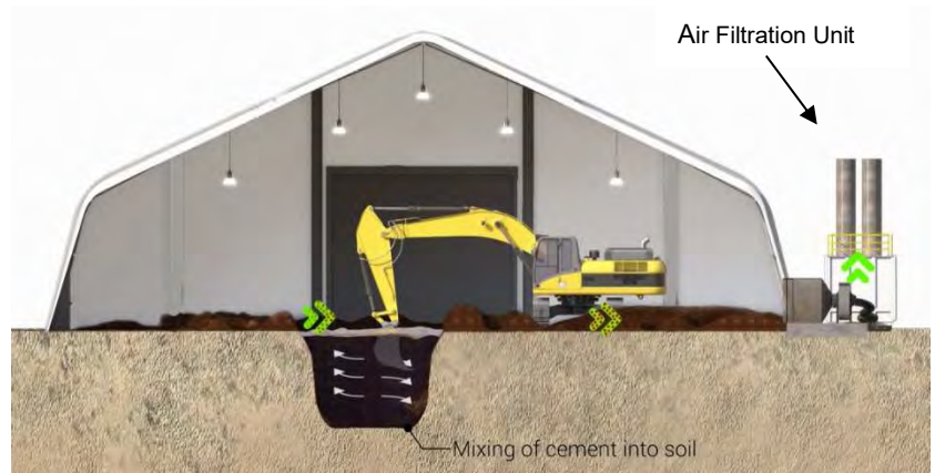
Soil solidification operations under tent
