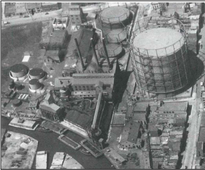
Manufactured Gas Plant at the Gowanus Canal
