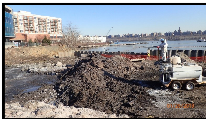
Worker applying Posi-shell.
