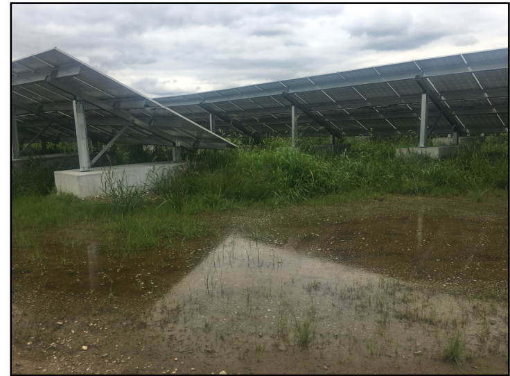
Photo 24. Ponding on northside of landfill, end of solar panel Row 1, facing southeast.
