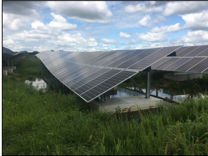
Photo 13. View of standing water in middle of solar panel rows, Row 25 facing northwest.
