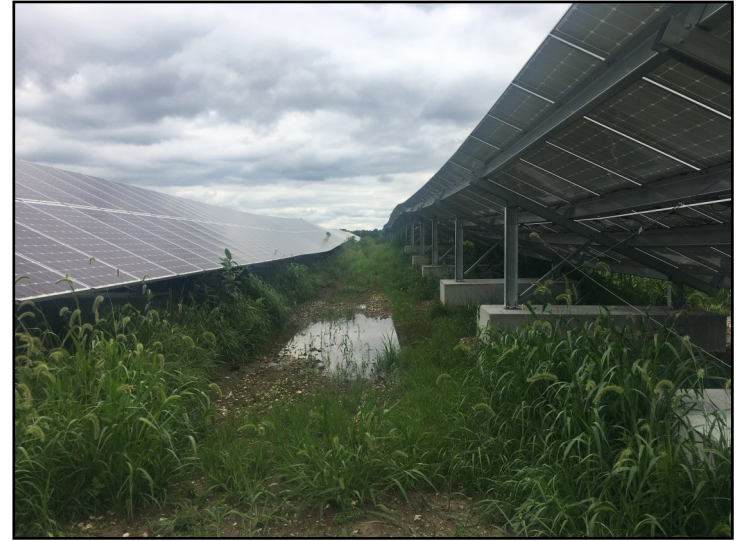
Photo 22. Typical ponding on westside of landfill, Rows 30-31.
