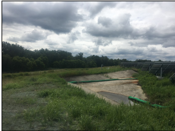
Photo 11. View of letdown channel on northeast corner, note iron staining from historical water seepage.
