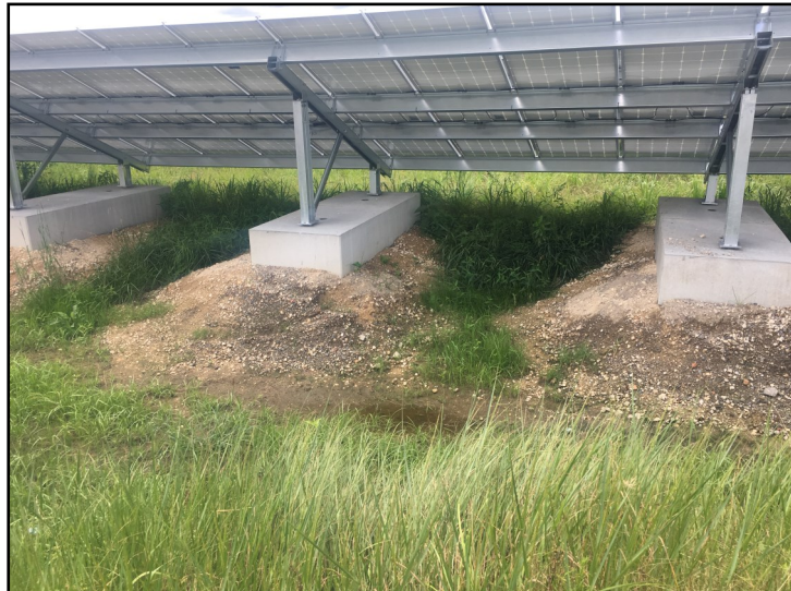
Photo 15. Example of small scale ponding and solar panel supports.
