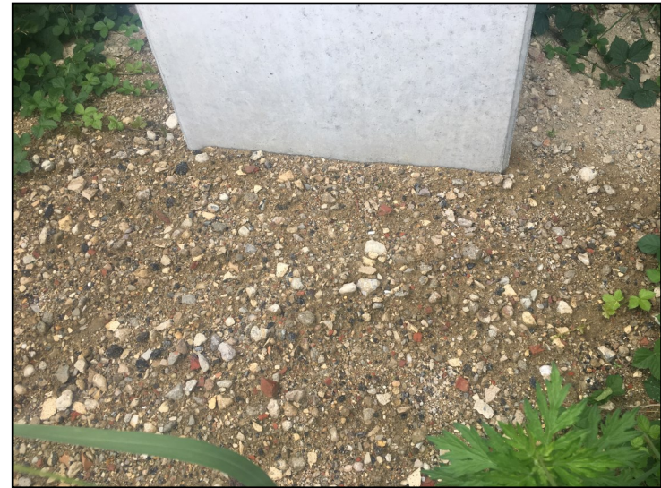
Photo 10. View of typical fill material used as base for solar panel concrete footers, note asphalt present.
