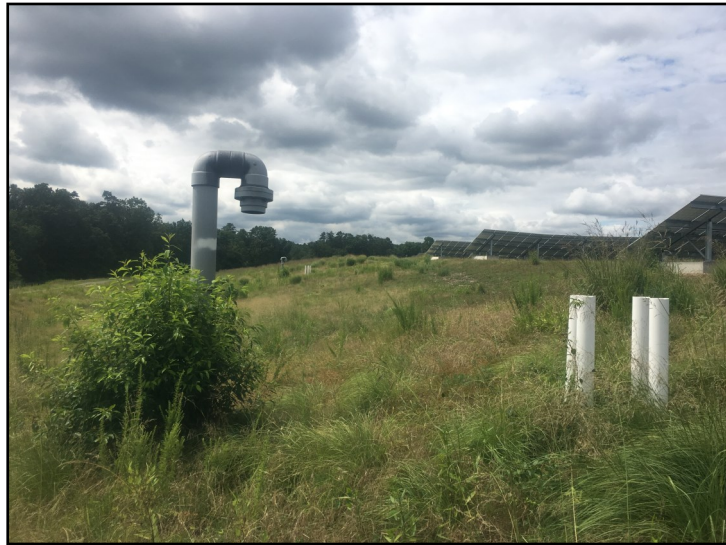
Photo 9. View of typical vent, note excess vegetation.
