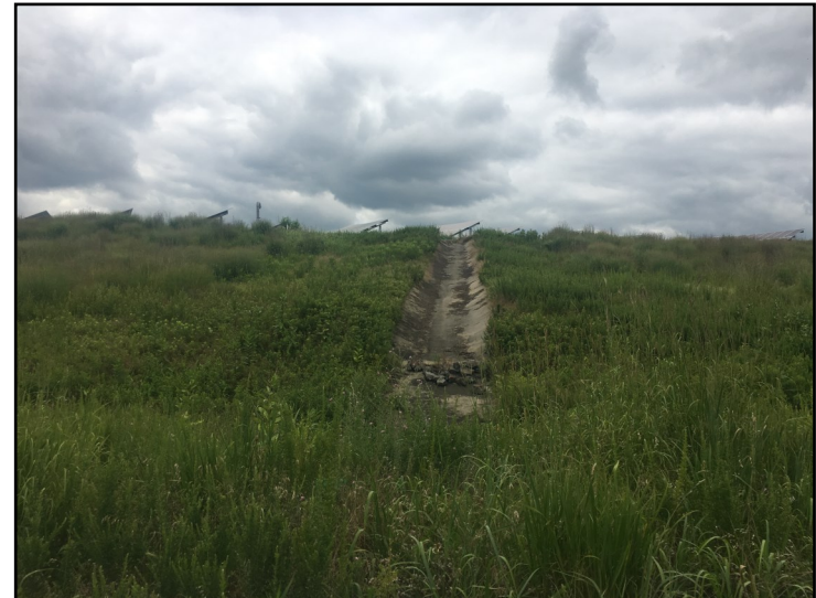
Photo 16. View of letdown channel east side of landfill facing west.
