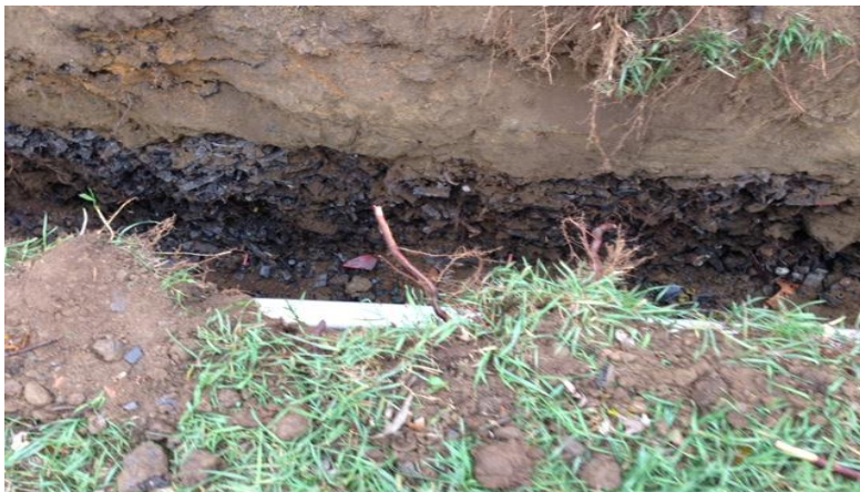
Figure 1: Buried crushed battery casings at Birchly Court
