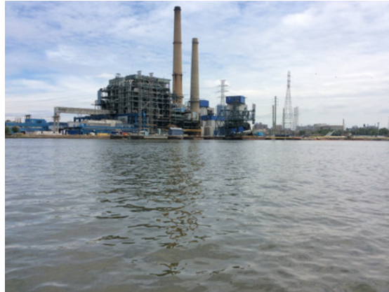
PHOTO LOCATION: HR-67.jpg DESCRIPTION: View to east of the power plant
