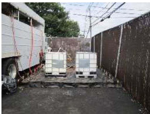
EVO in Secondary Containment
