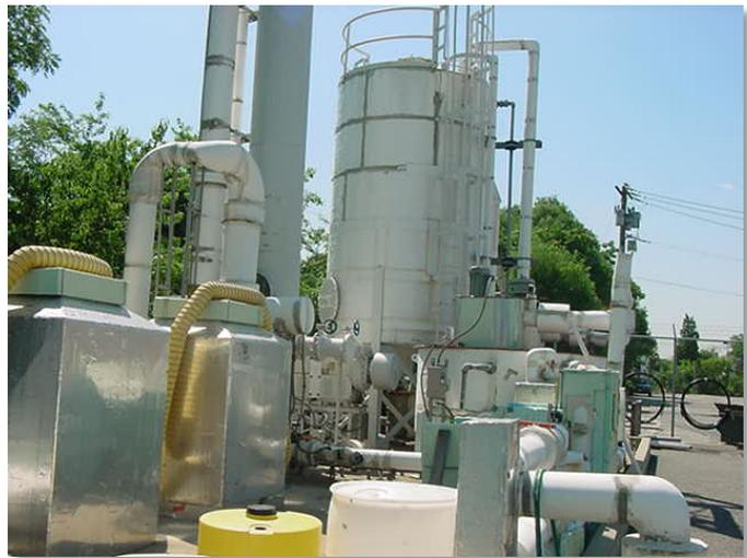
Figure 2. The groundwater remediation system, which extracted, treated and reinjected groundwater as part of the remedy at the Site.
