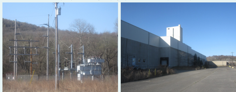
Electric substation (left); Building 5 (right); Warehouse (bottom)
