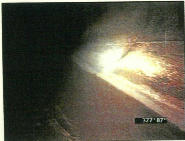
IMAGE: 14a, TAPE #: 01, 00:00:00 377.55FT, pipe
