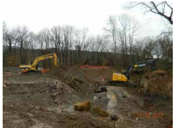
Excavation of Former Building 54 Area Soil for Slope Area Mitigation
