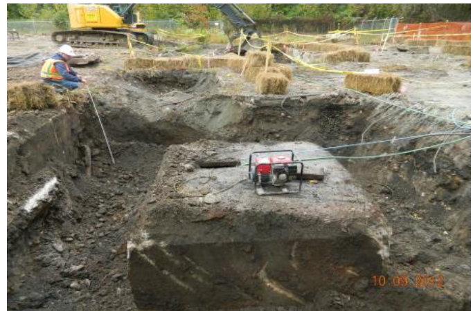
Unearthed Concrete Vault/Structure Located within TSCA #4 Location - Removal is Pending
