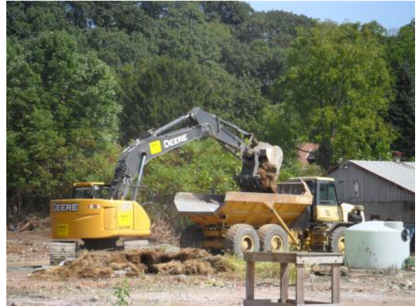
Transporting Former Building 57 Area Excavated Soil to Temporary Staging Area
