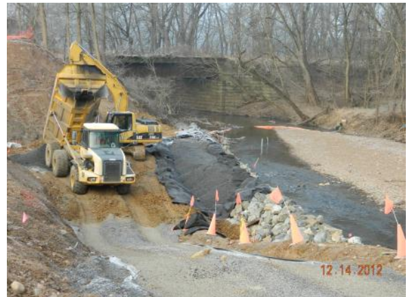
Loading TSCA Waste for Off-Site Disposal
