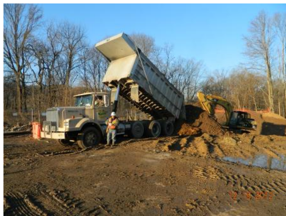
Receiving and Placing Imported Backfill
