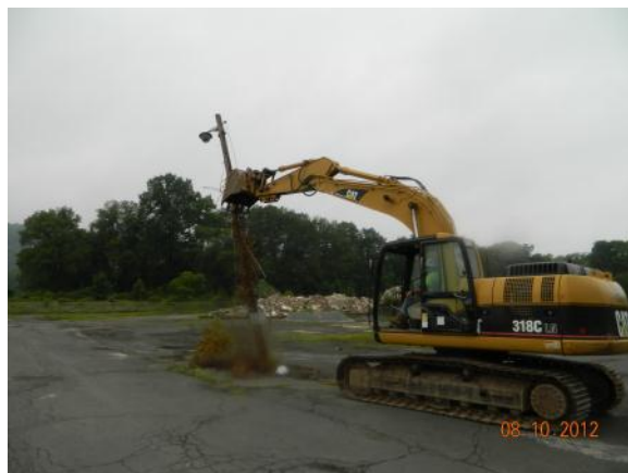
CFA Inactive Utility Pole Removal – Clearing Work Area
