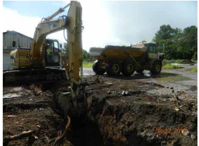
Removal of Underground Pipe DP-15
