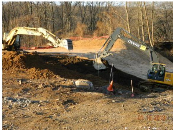
Backfilling Former Building 54 Area
