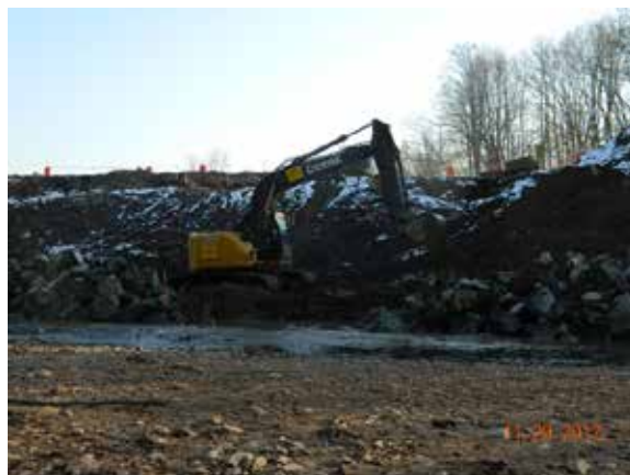
Completion of Rip-Rap Placement to Reconstruct Q Creek Embankment
