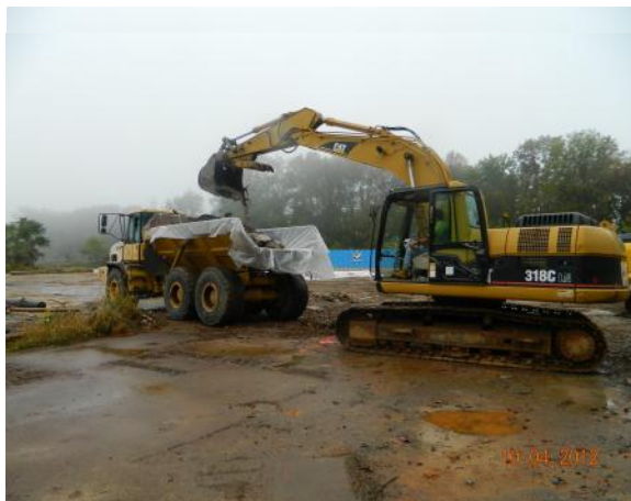
Loading Excavated Sump Area Soil for Onsite Staging
