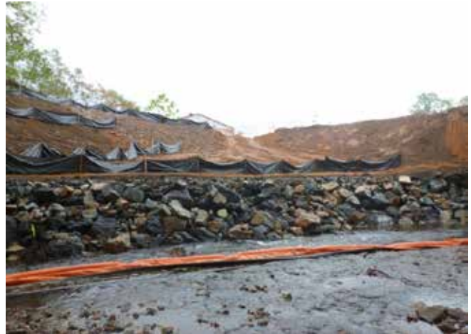
Fill and Topsoil Placed and Compacted at Former Building 57 Area
