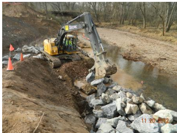
Placement of Stone Along Q Creek within Former Building 54 Area
