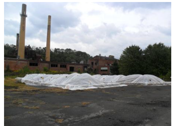
Lined Soil Staging Area
