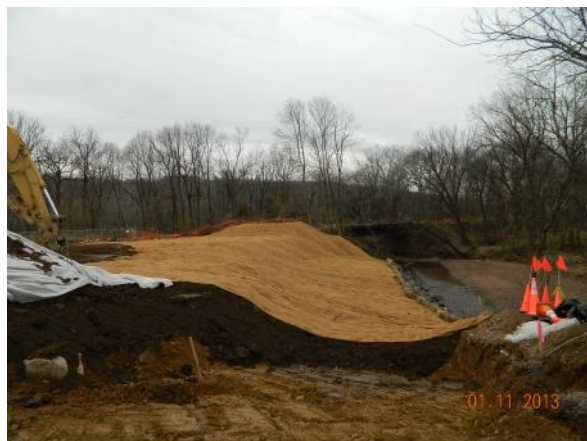
Former Building 54 Area Erosion Control Matting Placement
