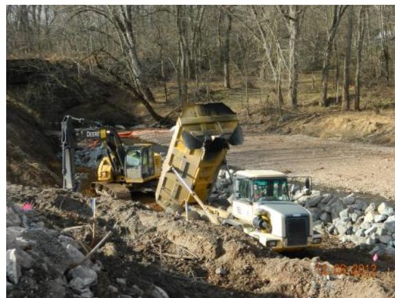
Backfilling Adjacent to Q Creek
