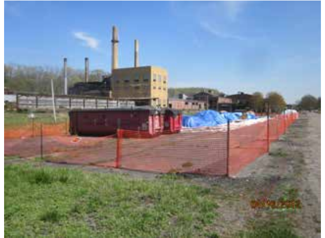
Heavier blue tarp utilized within MHLA to increase stability against heavy winds
