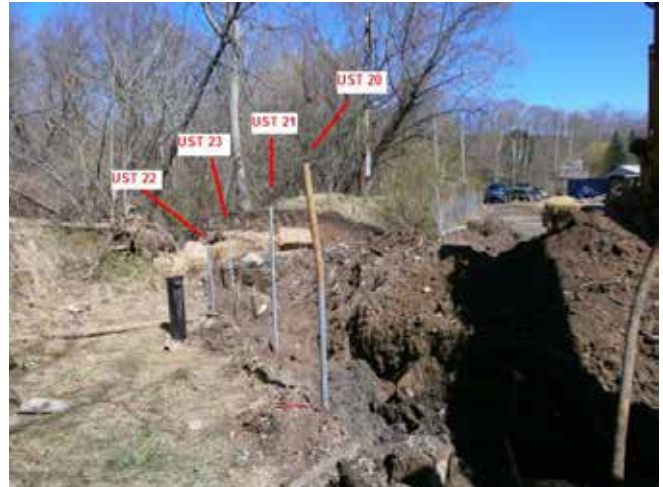
Test pits to locate USTs
