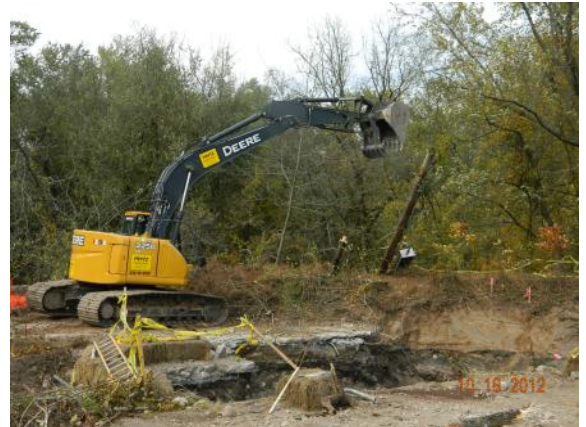
Former Building 54 Area Slope Mitigation Upper Soil Removal
