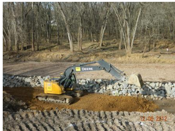
Continued Backfilling Adjacent to Q Creek
