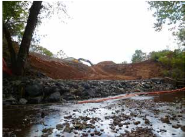
Completed Stone Placement Along Bank of Q Creek Former Building 57 Area
