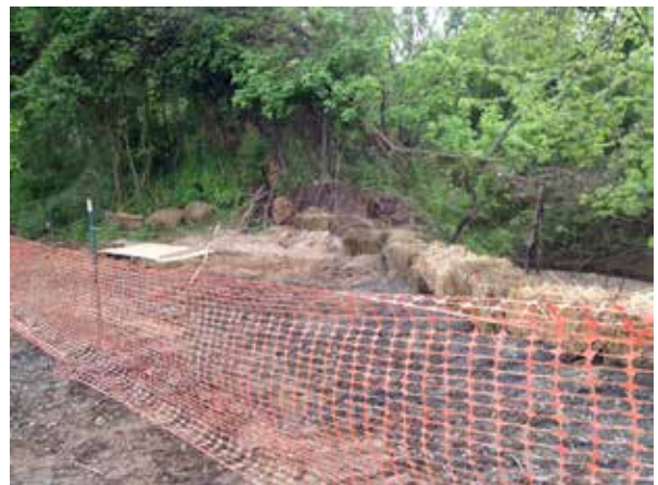
Restored excavation after removal of UST Nos. 22, 23, and X
