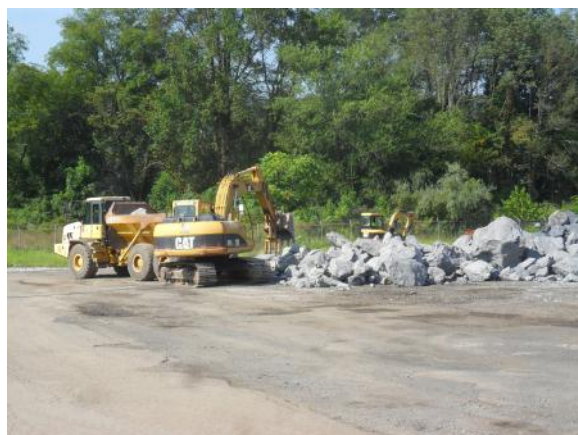
Staging Imported Stone for Q Creek Bank Restoration
