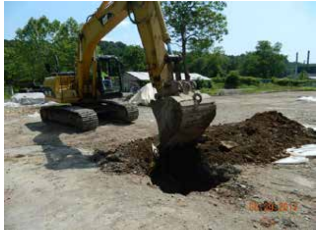
Test pit excavation
