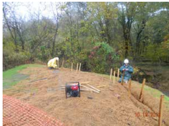
Former Building 57 Area Fiber Log Installations
