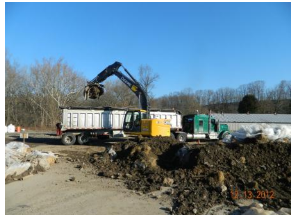
Loading TSCA Waste for Off-Site Disposal
