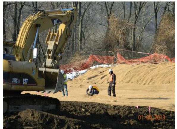
Installing Erosion Control Matting Over Seeded Topsoil
