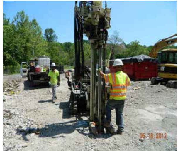
Soil boring installation
