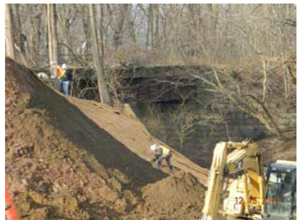
Former Building 54 Area Q Creek Embankment Reconstruction – Stone Placement
