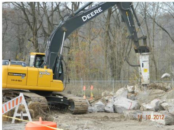
Sizing Concrete Excavated from UST #14 & #15 Area
