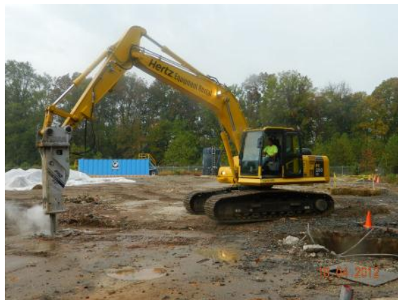
Concrete Removal – Former Building 54 Area Excavations
