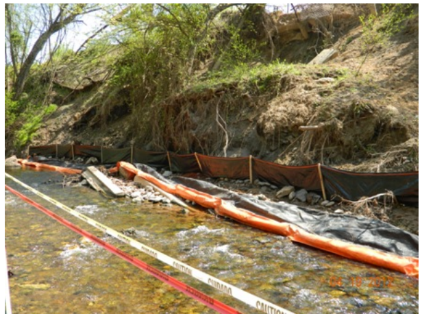
Silt Curtain installed within Q Creek, Silt Fence installed at toe of embankment adjacent to Q Creek
