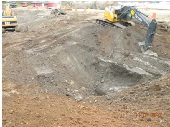
Soil Excavation from UST #14 & #15 Area
