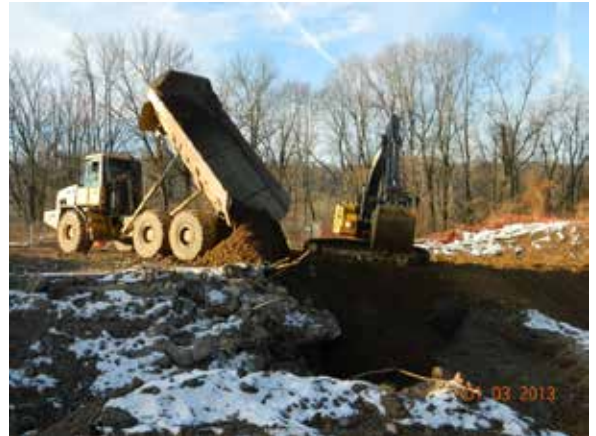
Backfilling Former Building 54 Area
