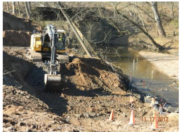
Excavation of Former Building 54 Area Soil Adjacent to Q Creek
