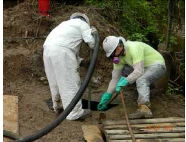
Vacuumping content of UST X
