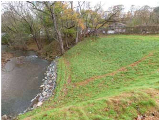
Former Building 57 Area Restored Slope – No Damage Observed Post-Hurricane Sandy
