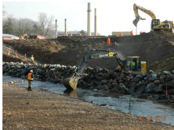
Rip-Rap Stone Placement – Q Creek Embankment
