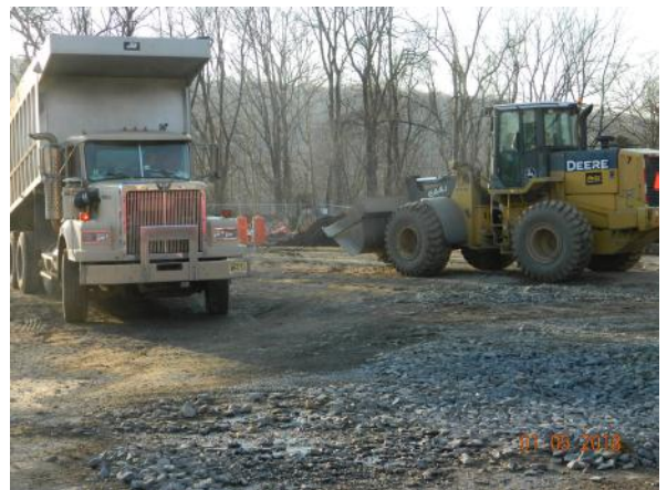
Handling of Fill for Backfilling
