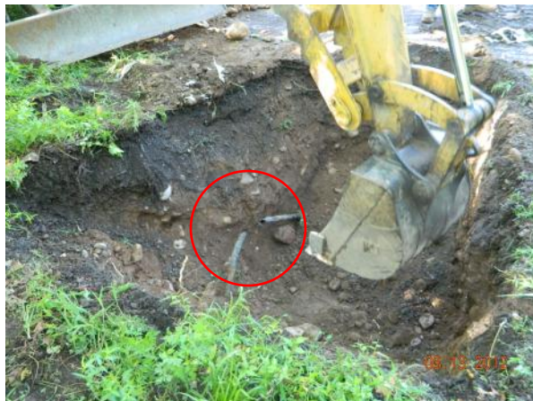
Excavation of test pit for investigation of unknown utility.
