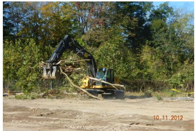
Former Building 54 Area Clearing & Grubbing – Preparation for Slope Excavation
