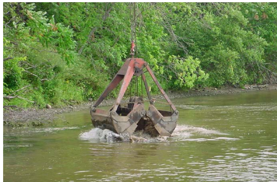
Photo: Capping Pilot Study - Cap Material Placement
