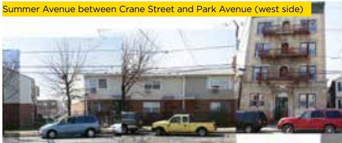
Summer Avenue between Crane Street and Park Avenue (west side)
