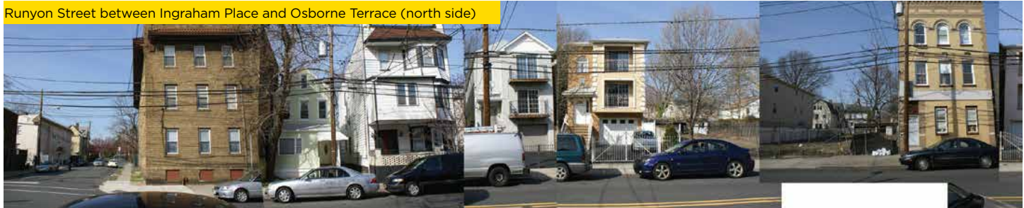
Runyon Street between Ingraham Place and Osborne Terrace (north side)
