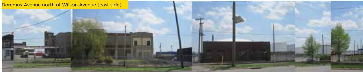
Doremus Avenue north of Wilson Avenue (east side)
