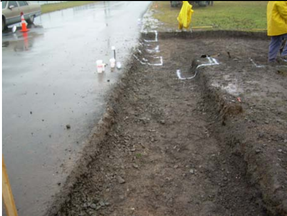
Picture 1: Sidewalk excavation and bollard layout
